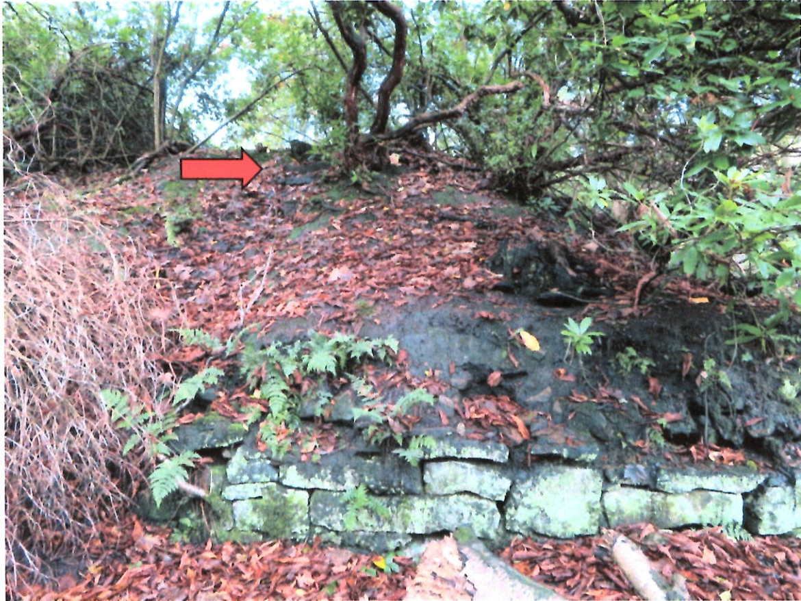
Plate 2 This raised bank appears to have been part of the bowling green. The steps can still be seen (arrowed)
