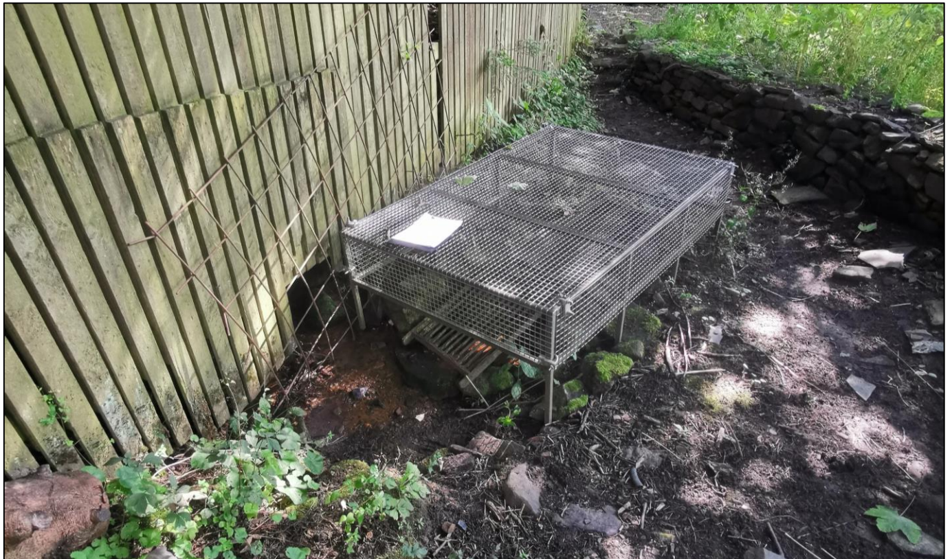
Figure 6 Ultimate Site culvert to the southeast corner.
