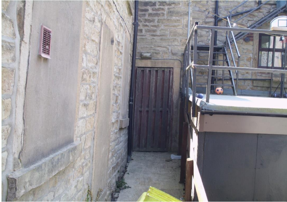
Existing service entrance to rear of No 6
