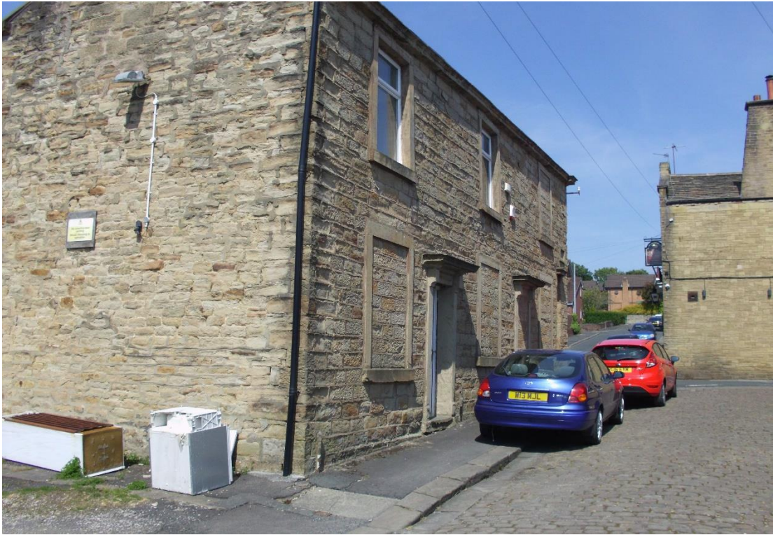
Havelock Street and Rear Gable End.
