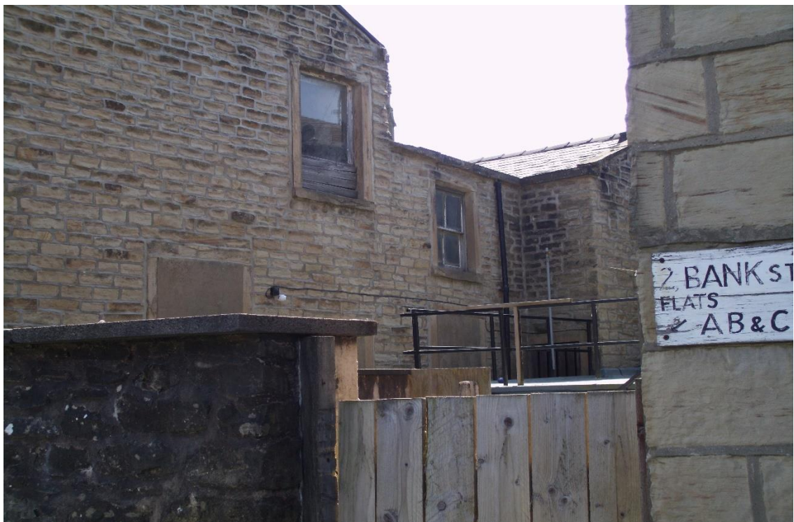
Side Facing North Street
