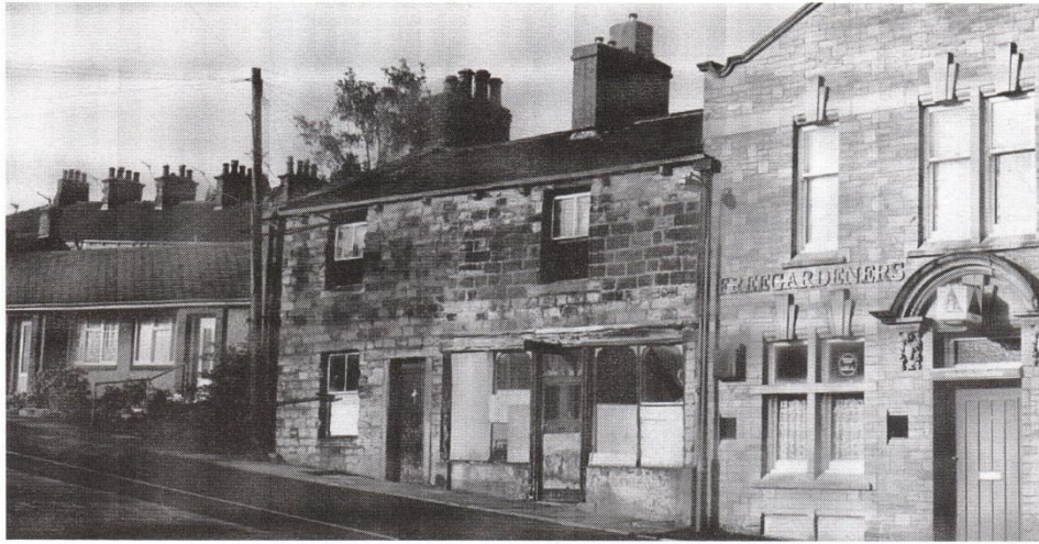
The Free Gardeners at 2 St Giles Street, seen here in 1983, is named after the United Order of Free Gardeners, a friendly society. Laurel Lodge, a Padiham branch of the Free Gardeners, was established in 1827. Sixty years before this photograph was taken, the building above the Free Gardeners was the busy grocer's shop belonging to Jimmy Hargreaves, but by the time this photograph had been taken it had recently been vacated by Alf Thompson, electrician. There was a strange incident at the pub which happened to
