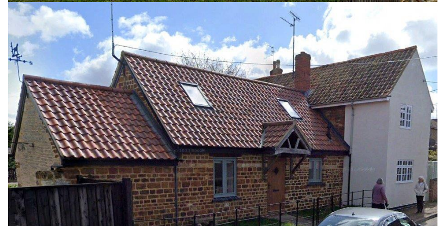
Figure 7 – Typical Materials (source: Google Streetview)
