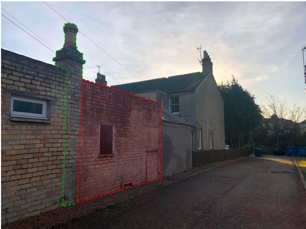
Figure 1. Rear elevation of existing outbuilding viewed from Kinnessburn Cottages. Portion to be demolished highlighted in red, shared chimney to be retained highlighted in green.
