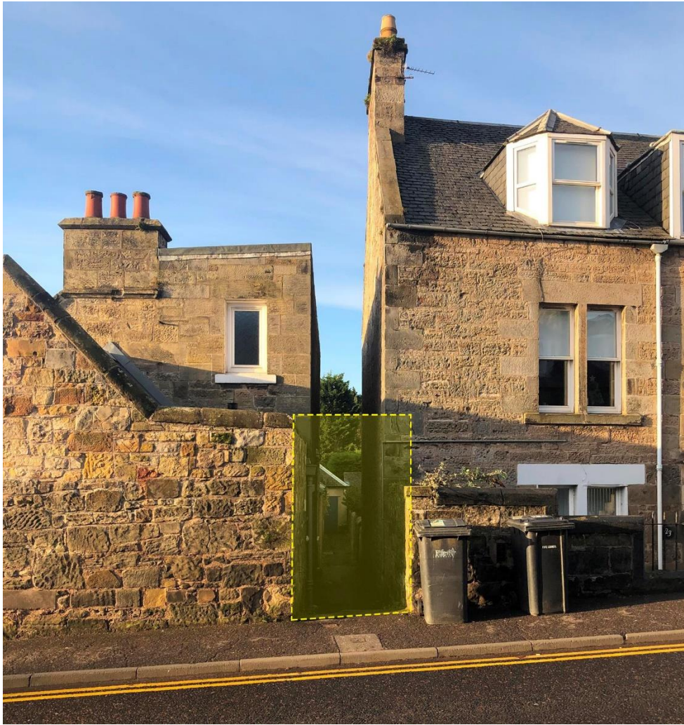
Figure 3. Existing access pend highlighted in yellow as viewed from Melbourne Place.
