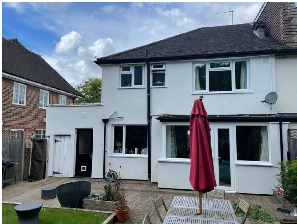
View of rear façade of house and patio
