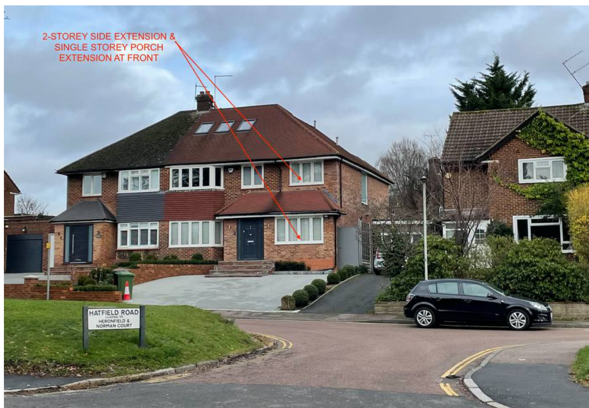
Front view of nearby no 81 Norman Court (EN6 1HZ) which has had a 2-storey side extension under an extended hipped roof and a single storey front extension with porch combined into one element. This is the general precedent which we are following for the front projection at no 61 Hatfield.
