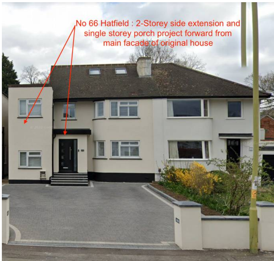
Front view of no 66 Hatfield road showing combined side and front porch extensions
