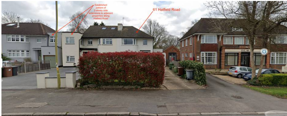
Streetscape view showing no 61 Hatfield Road in the context of adjacent two-storey & one-storey side extensions and front extensions
