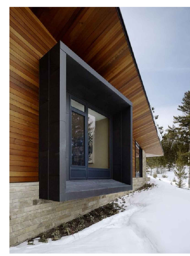
Stained Cedar Reveals
