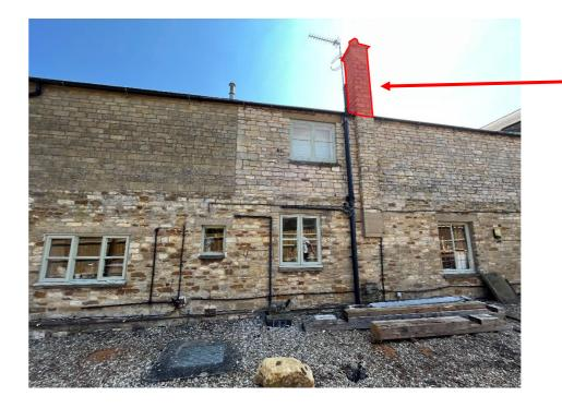
Limestone stack reduced down to eaves level, below the gutter line. Guttering adapted to sail over the remaining protrusion.
