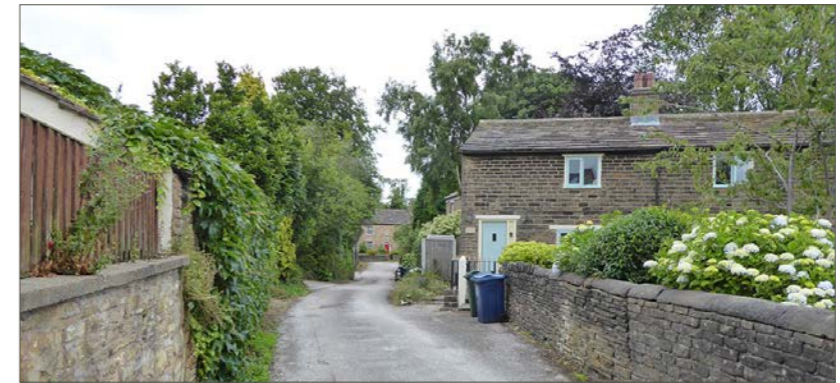
Traditional stone cottages and boundary walls, north of both the Plough and Harrow pub, Ormskirk Road
