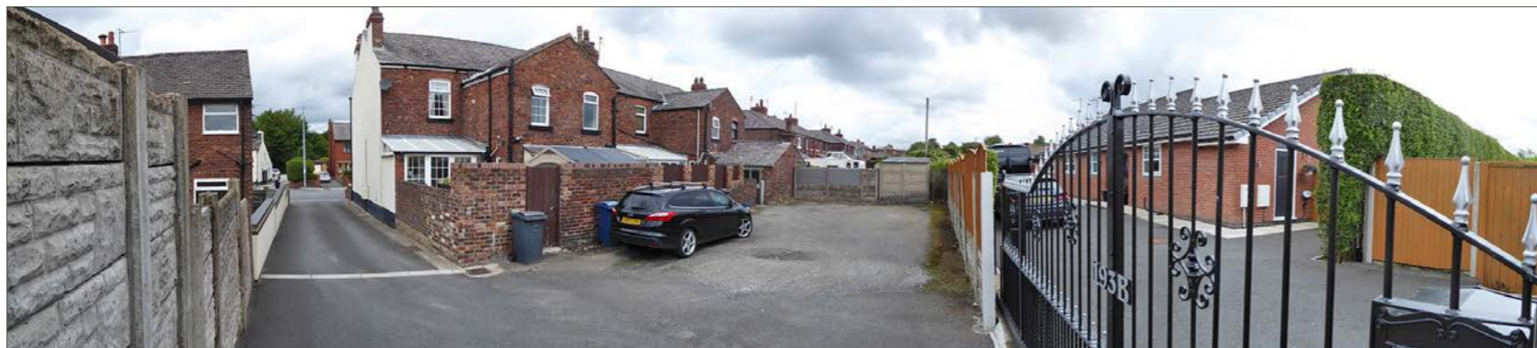
Access to 193b Ormskirk Road and rear parking area serving 195-203 Ormskirk Road between 201 and 203 Ormskirk Road
