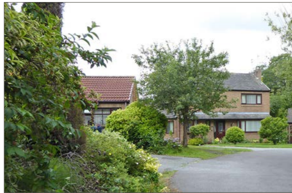
1980's detached development to the north of Ormskirk Road finished in buff / brown brick
