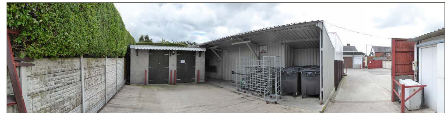
Far eastern site boundary defined by a concrete panelled retaining wall with dense hedgerow / vegetation above
