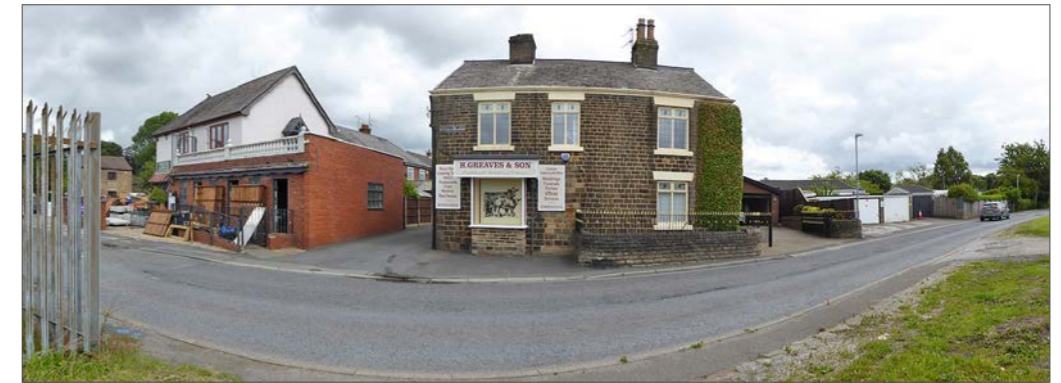
The rendered Venilde and Sons Ltd. corner premises and rear extension with balustrade alongside the existing site access to both the previous butcher's yard and main commercial area
