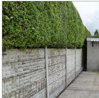
Far eastern site boundary. Proposals will be separated visually by a circa 1.75m high concrete panel retaining wall, with dense hedgerow above.
