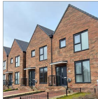
Design cue and thoughts around housetypes and typology development. Alternating brick bonds adding texture and variety
