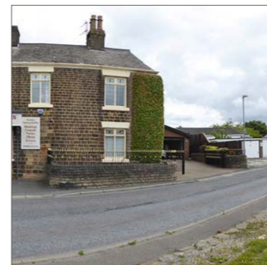
Existing southern access to 1-3 Chequer Lane
