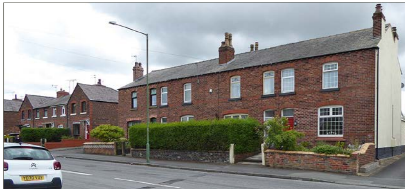
Attractive / more traditional red brick 19 th Century residential terrace with brick string coursing and detail, arched window heads and chimneys at 195-201 Ormskirk Road
