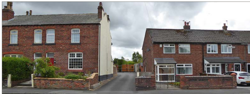
Access to 193b Ormskirk Road and rear parking area serving 195-203 Ormskirk Road between 201 and 203 Ormskirk Road
