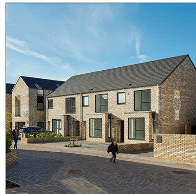
Design cue - contemporary units with large anthracite openings and good quality buff brick
