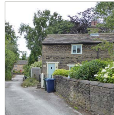
Traditional stone cottages and boundary walls, north of both the Plough and Harrow pub, Ormskirk Road
