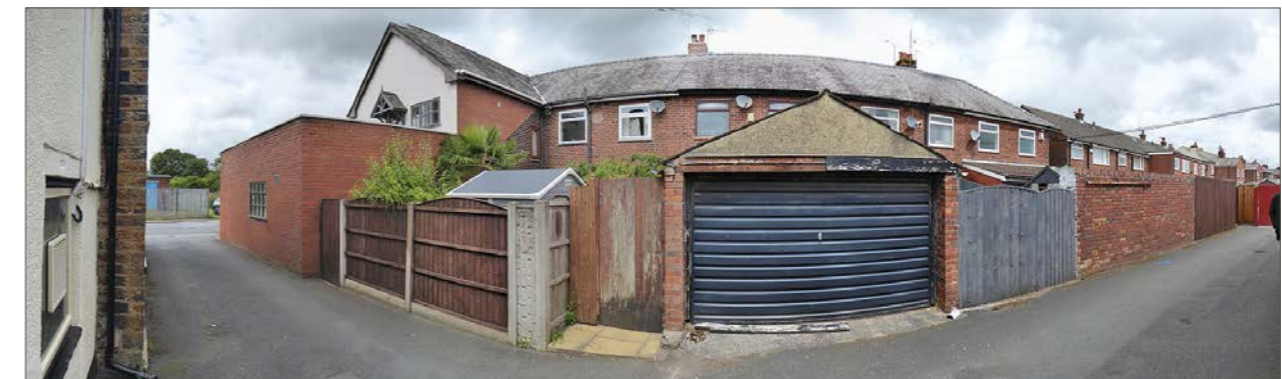
Irregular plot fencing and walls, various flat and pitch roofed sheds / outbuildings, and a single pitch roofed garage serving No217 Ormskirk Road make up initial elements of the site's north westernmost boundary
