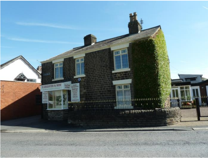
Photograph 1: – B1 general view front elevation.
