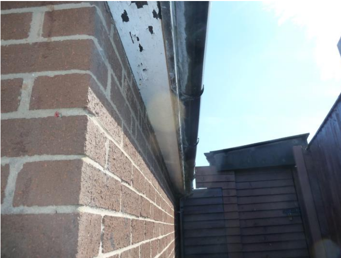
Photograph 33: - B3 south elevation with entrance to covered passageway visible. (See photo 29)
