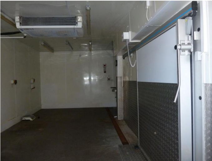
Photograph 26: - B2 internal view of food preparation and storage areas.
