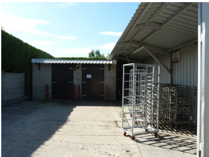
Photograph 23: - B2 general view of construction type of outdoor storage area. austere, single-skin, no gaps or void spaces.
