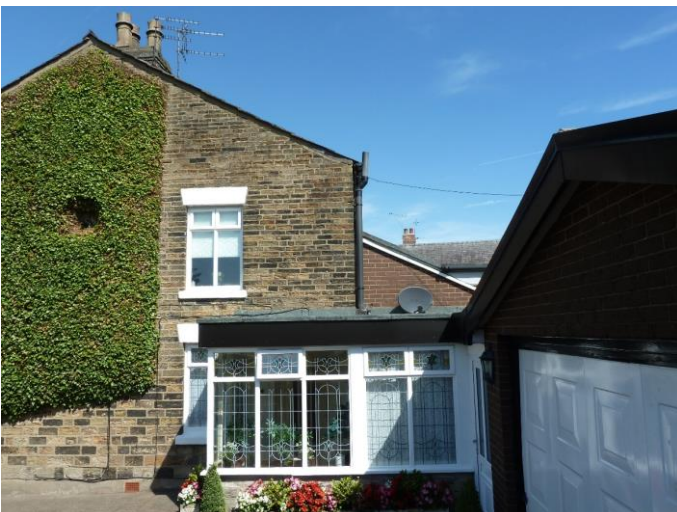
Photograph 3: – B1 General view – south gable elevation.
