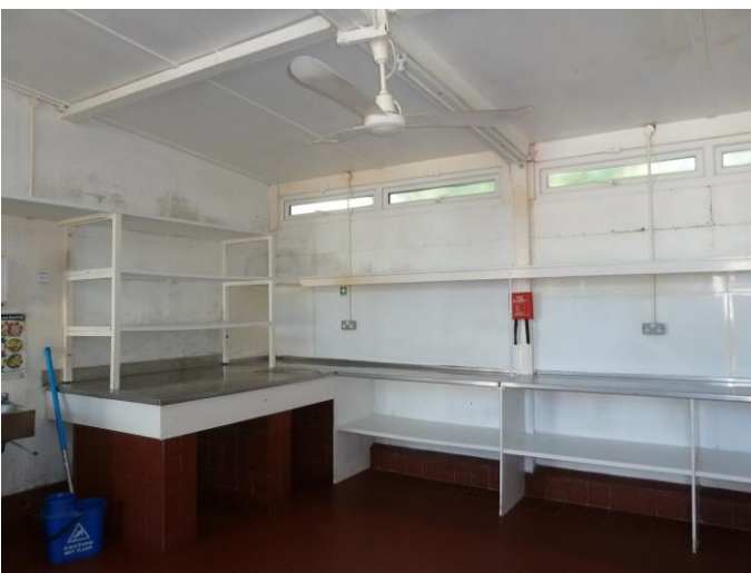
Photograph 27: - B2 internal view of food preparation and storage areas.
