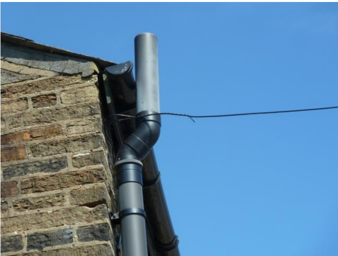
Photograph 5: – B1 corner of south gable and east elevation – wide gap behind fascia board.
