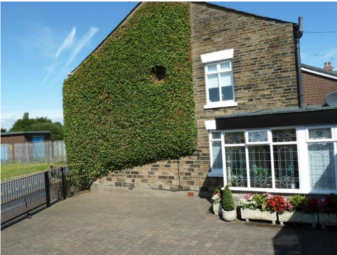
Photograph 2: – B1 General view – south gable elevation.
