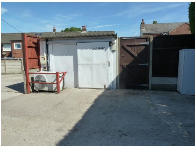
Photograph 22: - B2 general view of construction type, austere, sealed units, no gaps.
