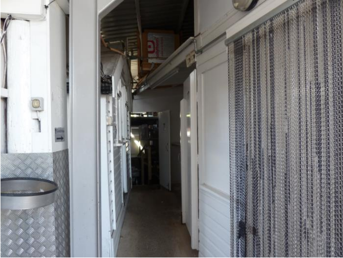
Photograph 28: - B2 internal view of food preparation and storage areas.
