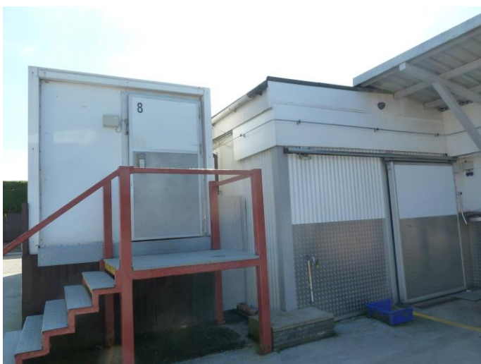
Photograph 24: - B2 general view of construction type – sealed units, no gaps or means of bat access.
