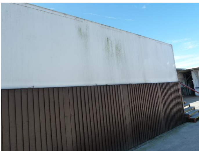
Photograph 20: - B2 general view of construction type, austere, sealed units, no gaps.
