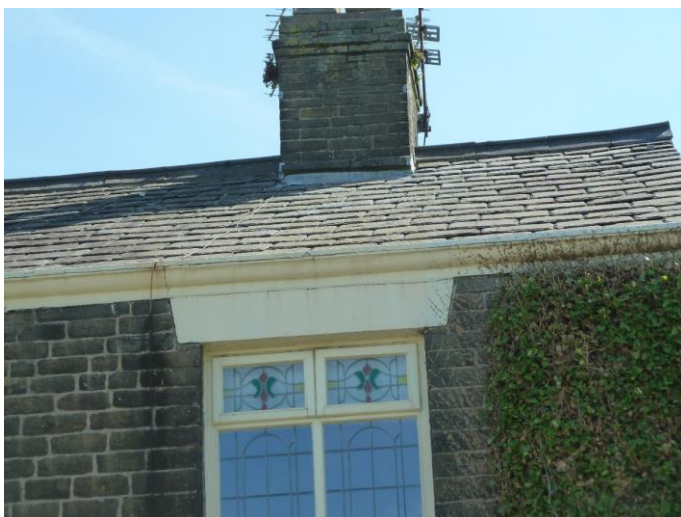
Photograph 8: – B1 general view of roof from across road.
