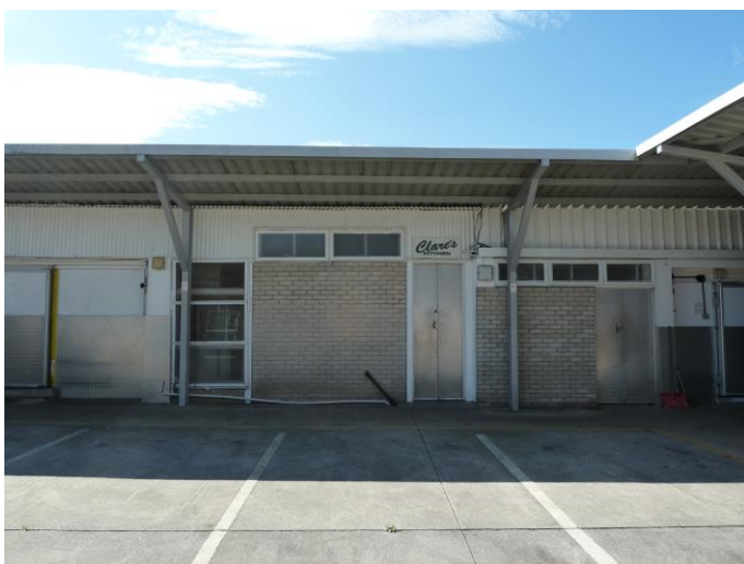
Photograph 17: - B2 general view of construction type of food preparation and storage areas.
