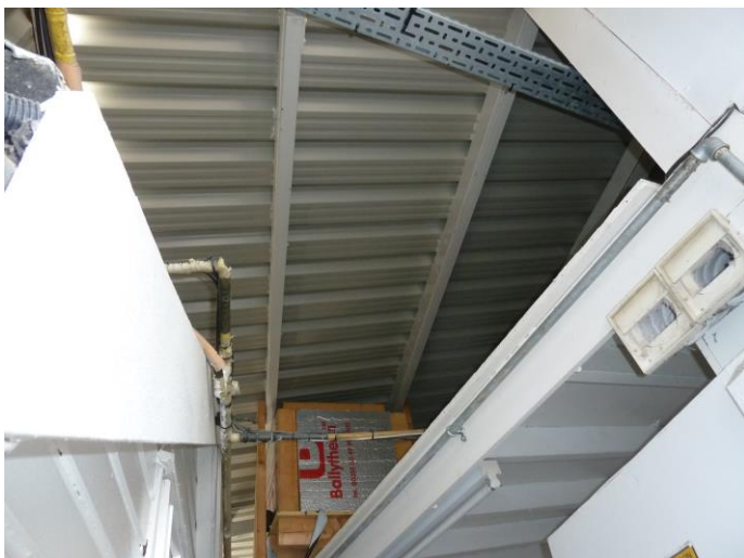
Photograph 19: - B2 general internal view of austere construction type.
