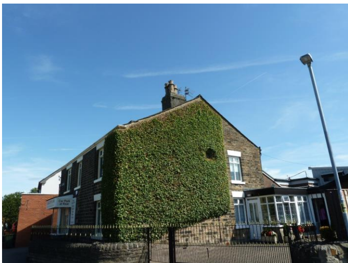
Photograph 7: – B1 general view – south gable elevation.
