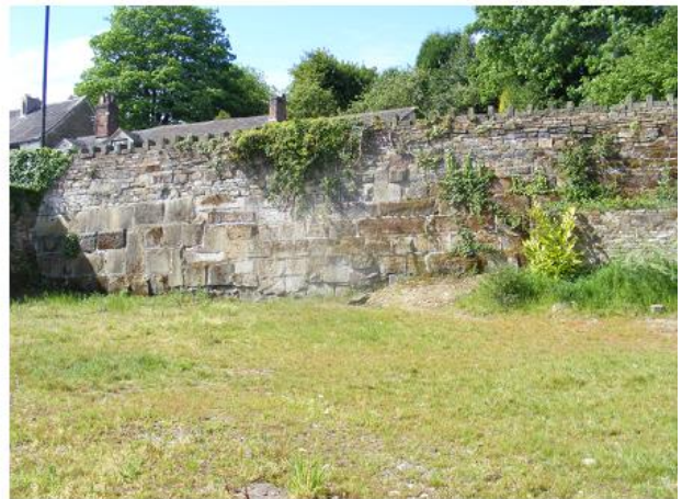
PHOTO 6 Eastern Elevation of Western Wall.
