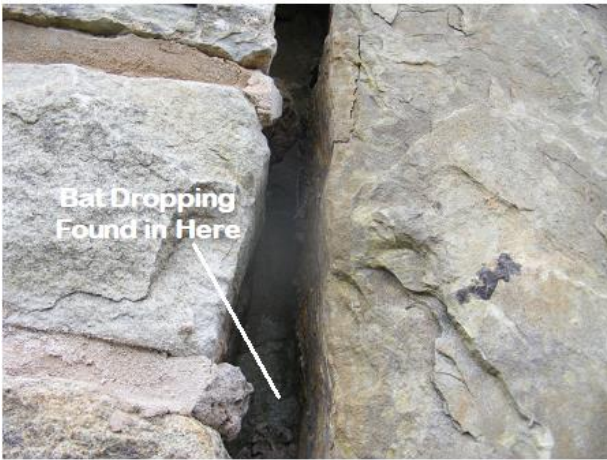
PHOTO 9 Central Expansion Joint
