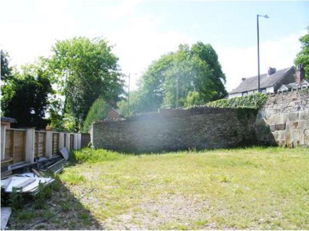
PHOTO 7 Northern Elevation of Southern Wall.
