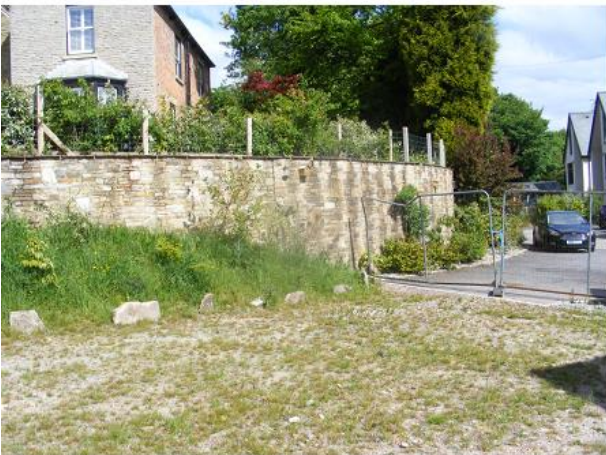
PHOTO 5 North-eastern End of Wall
