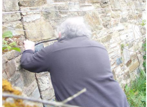
PHOTO 12 Surveyor with Endoscope at Eastern Joint
