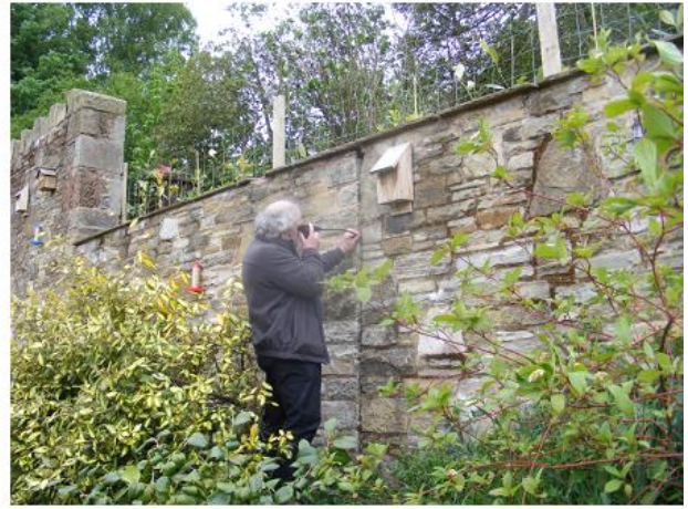
PHOTO 10 Surveyor with Endoscope at Central Joint
