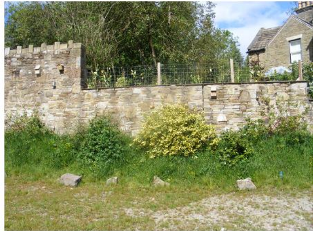
PHOTO 4 Central Southern Elevation of Wall
