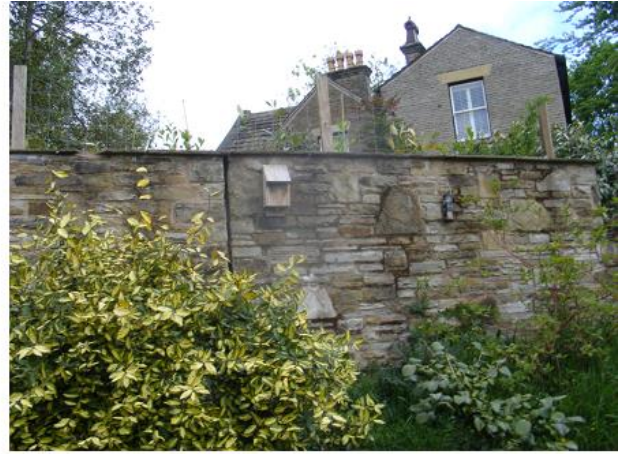
PHOTO 8 Southern View of Central Expansion Joint
