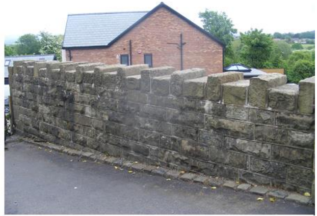
PHOTO 2 Northern View of Western End of Wall
