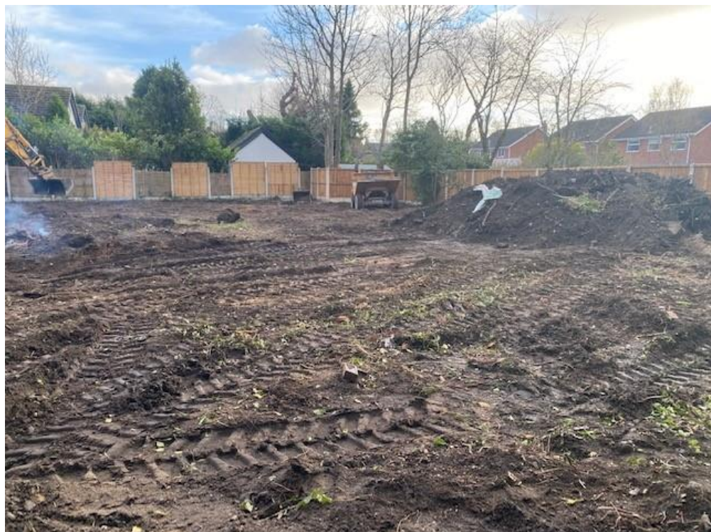
View toward the South West Corner of the site
