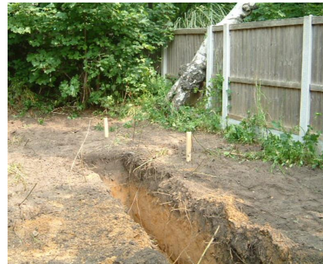
PHOTO OF EXCAVATED FOUNDATION
