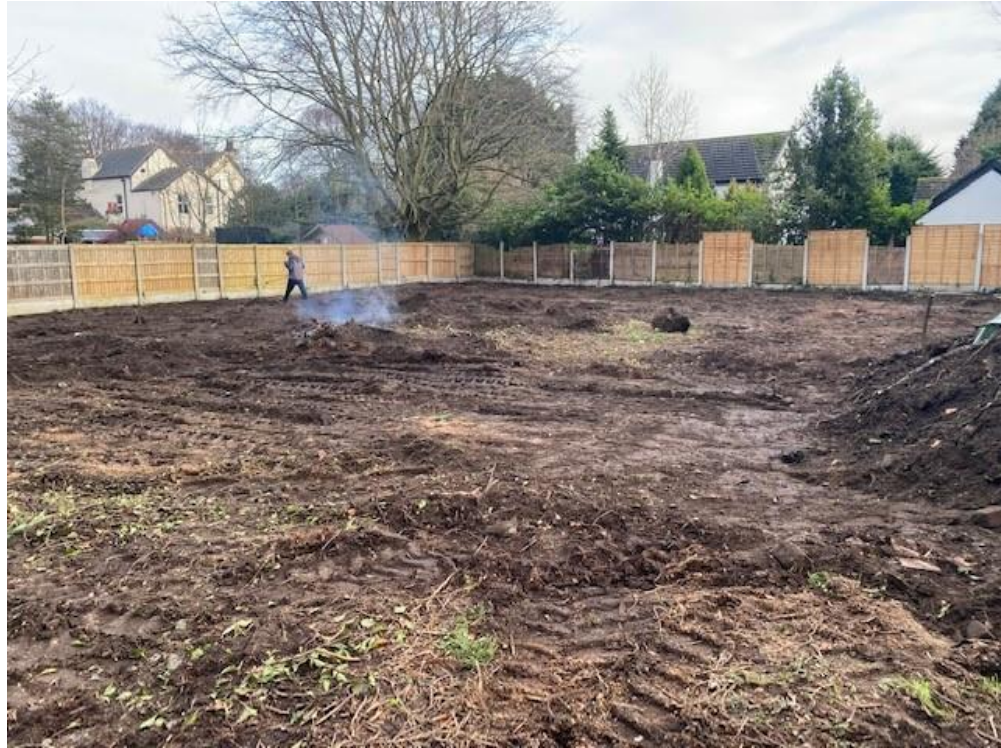
View towards the South East Corner of the site
