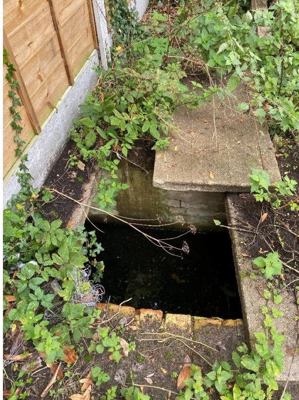
Plate 9: Open drain at south of site
