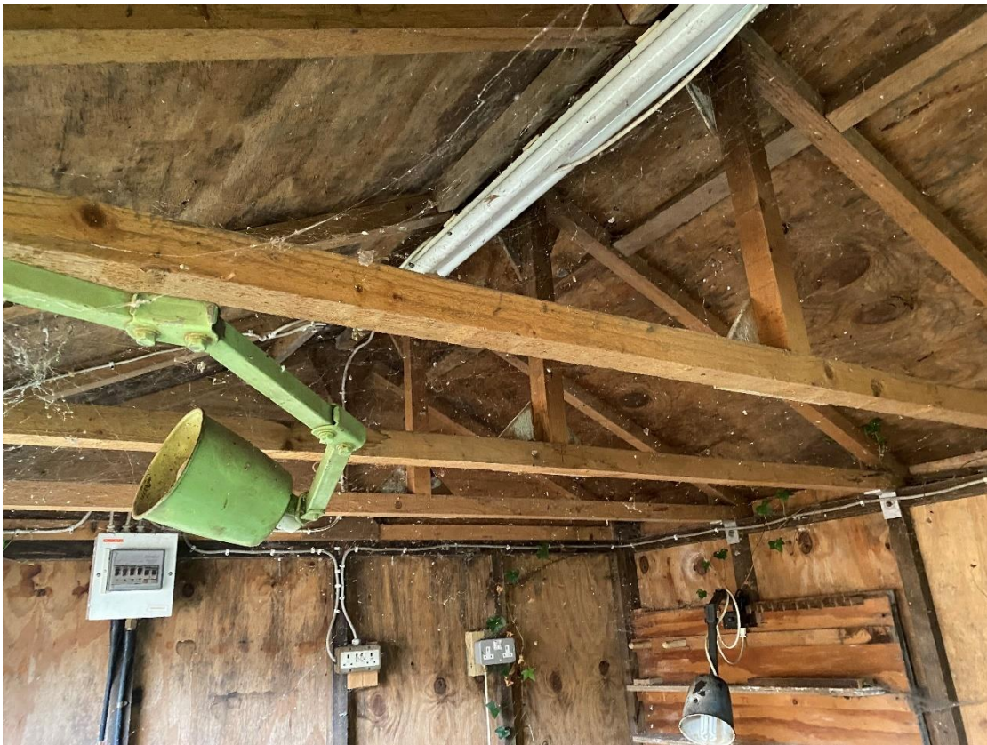
Plate 8: Internal character of shed continued
