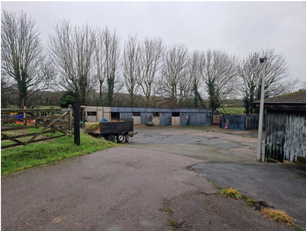
Existing Stables and Outbuildings.
