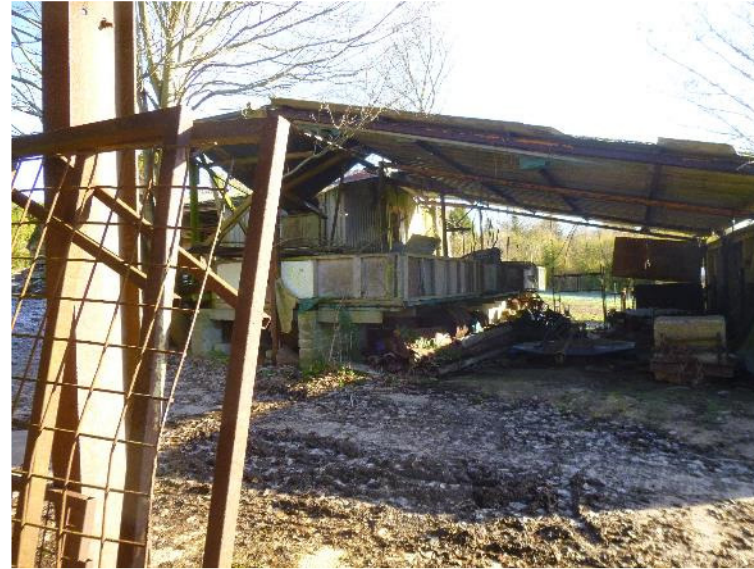
Fig.8.0 – Photograph showing building 8 with its covered hardstanding storage area.
