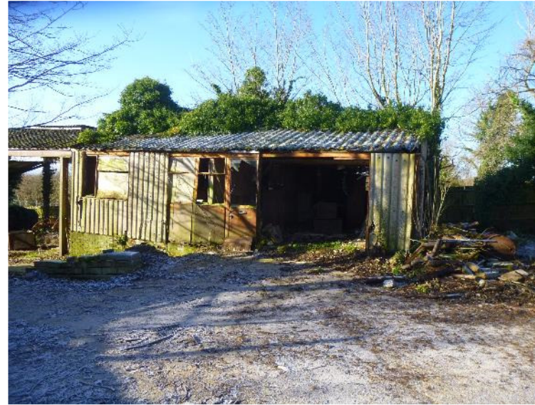
Fig.2.0 – Photograph showing existing building 4. Note the hardstanding to the front.
