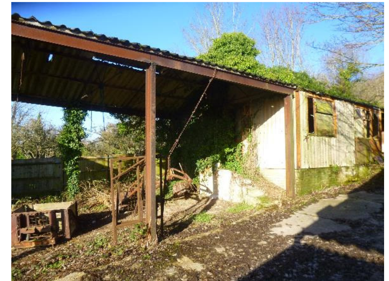
Fig.3.0 – Photograph showing existing building 4. Note the hardstanding to the front.
