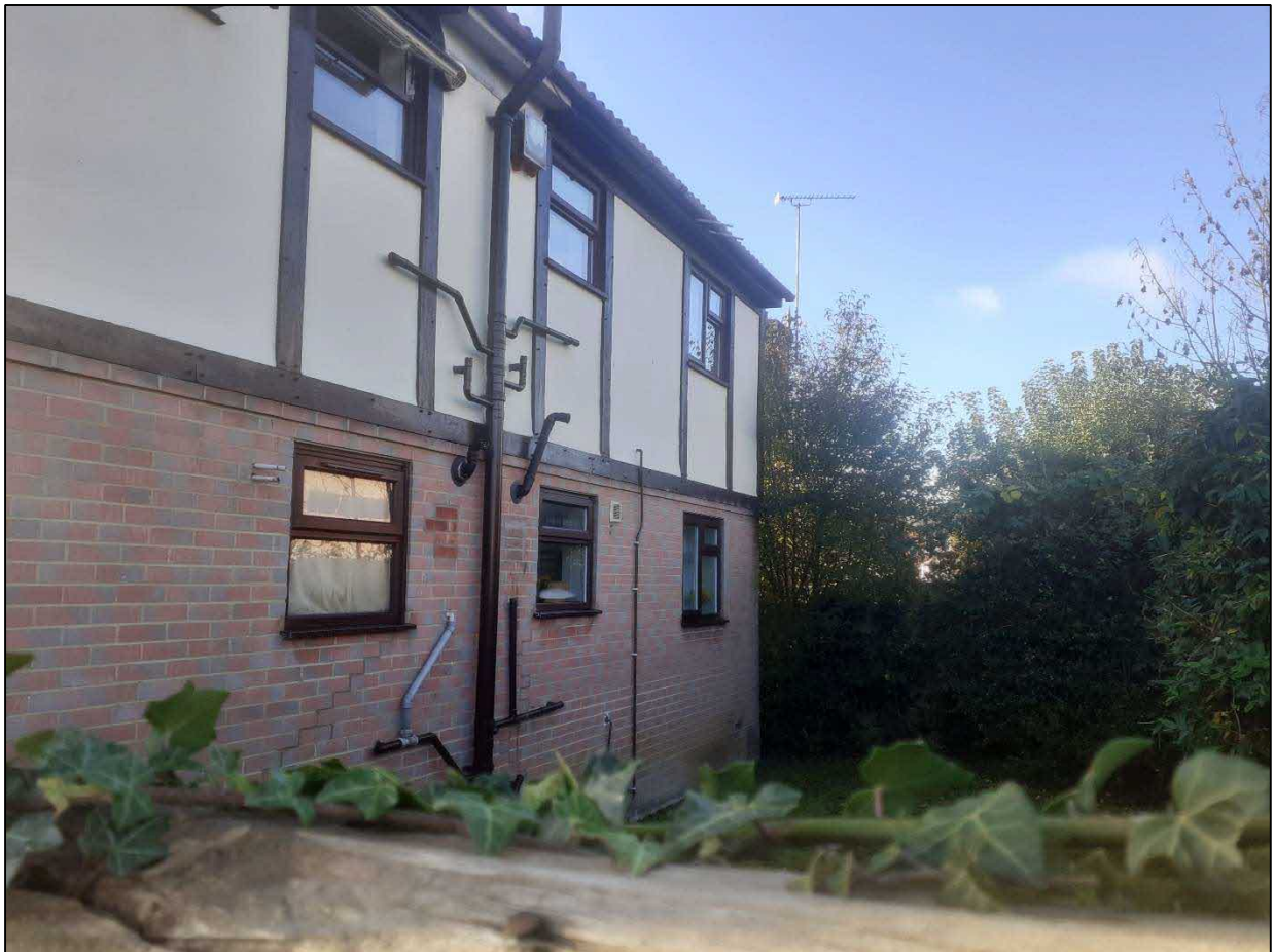
Figure 11: Rear elevation of Willow House.
