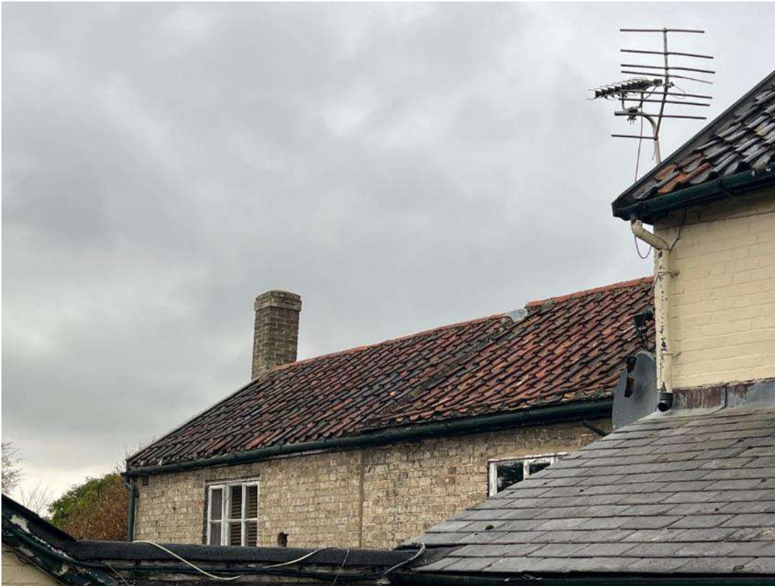
Photo 14. Building section 3 (ref B3A). East aspect of building.
