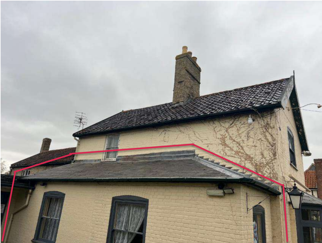
Photo 9. Building section 2 (ref B2A and B2B). Shows evidence of climbing plant on side of section B2A. Section B2B is identified by the red outline.
