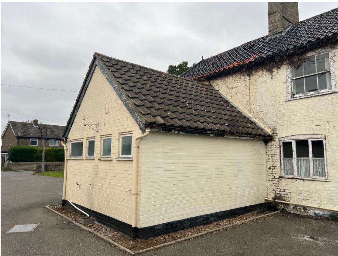
Photo 2. Building section 1. Rear of building, adjoining to building section 2 (ref B2A).
