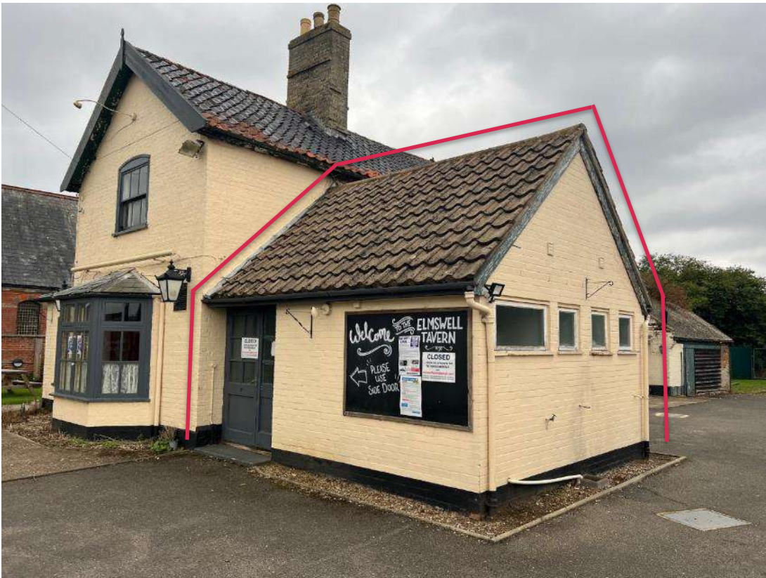
Photo 1. Building 1 as outlined in red. North east aspect.
