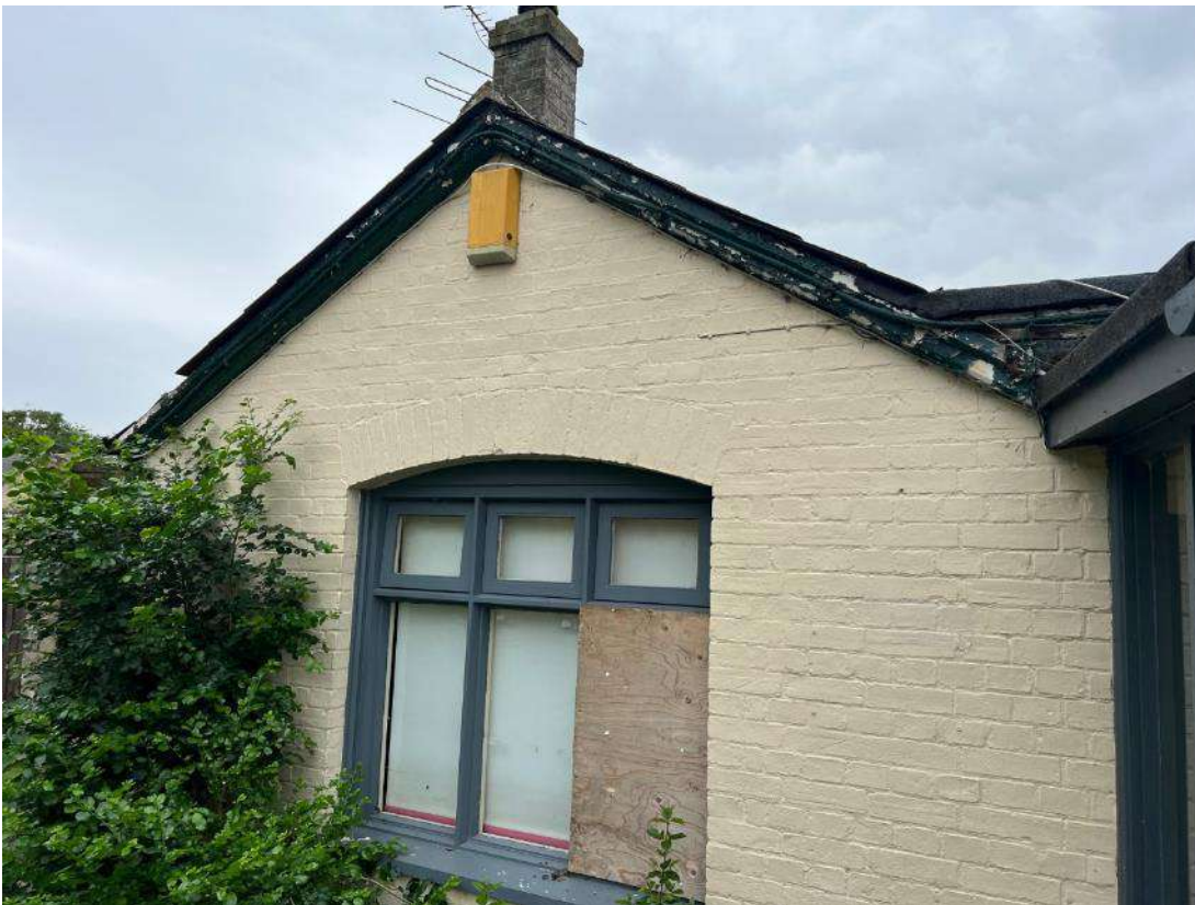
Photo 28. Building section 5. Shows northern gable end.
