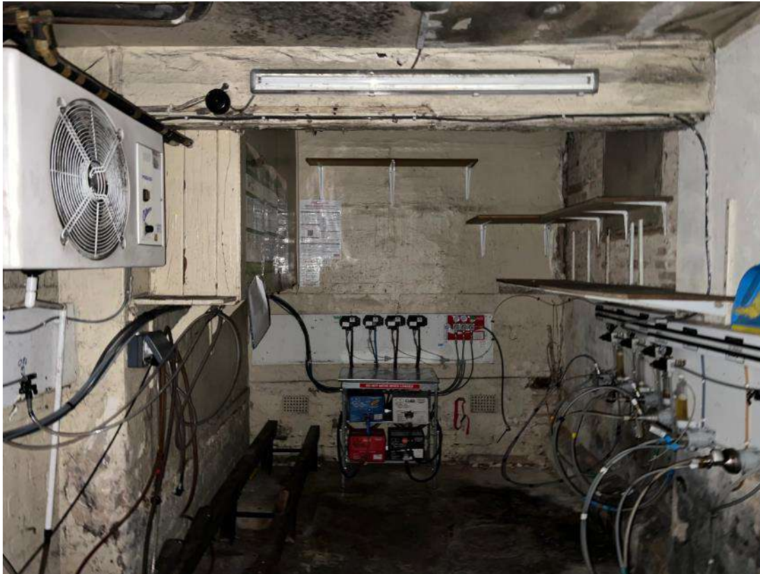
Photo 31. Cellar at base of building 3. Looking south.
