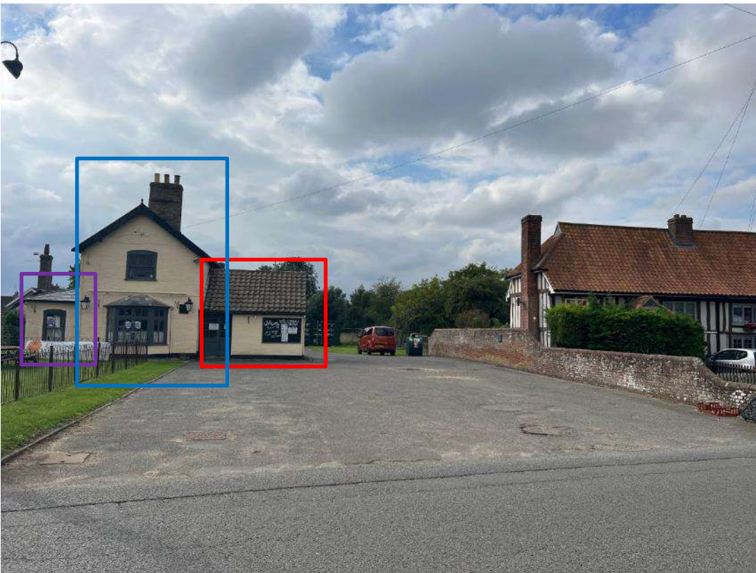
Photo 36. Taken from the road, looking at extensive area of tarmac, providing access and parking for the tavern. Grassland area 1 along with metal railings are also shown. Section 1 is shown in red, section B2A is shown in blue and section B2B is shown in purple.
