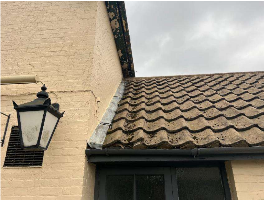
Photo 3. Interface between building 1 and building 2. Gap under lead flashing. Shows most of gaps under pantiles as being infilled with mortar. All gaps here, were cobwebbed.
