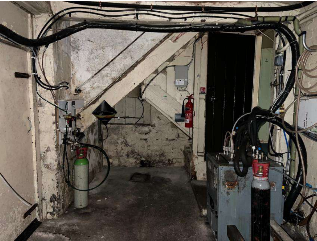
Photo 30. Cellar at base of building 3. Looking north.
