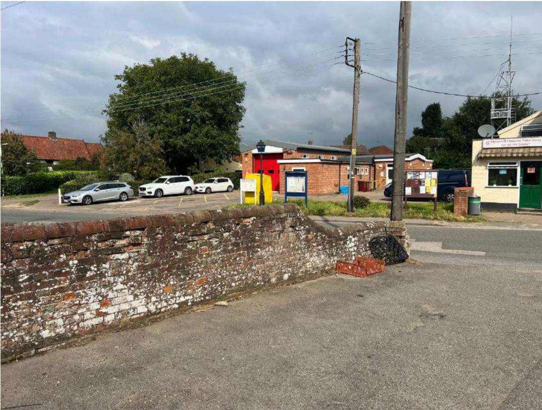
Photo 37. Shows brick wall along north west corner of site alongside road.
