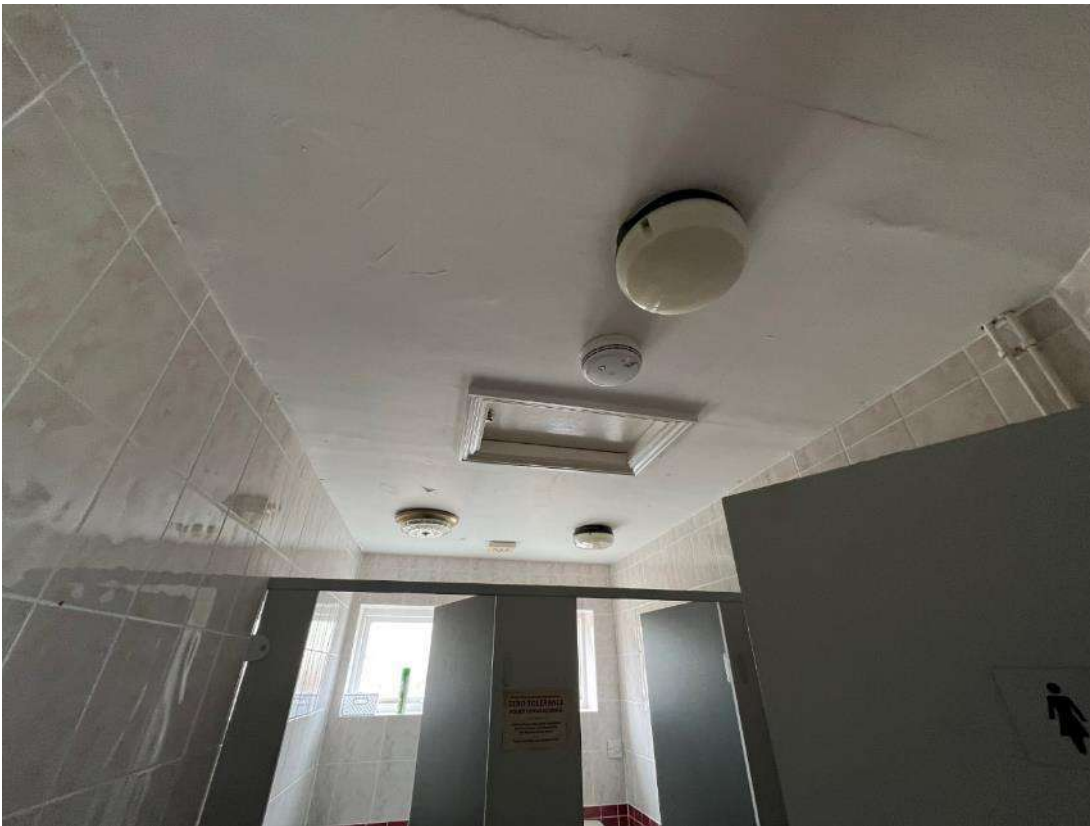
Photo 5. Building 1. Shows access hatch to roof space, within ladies toilets.
