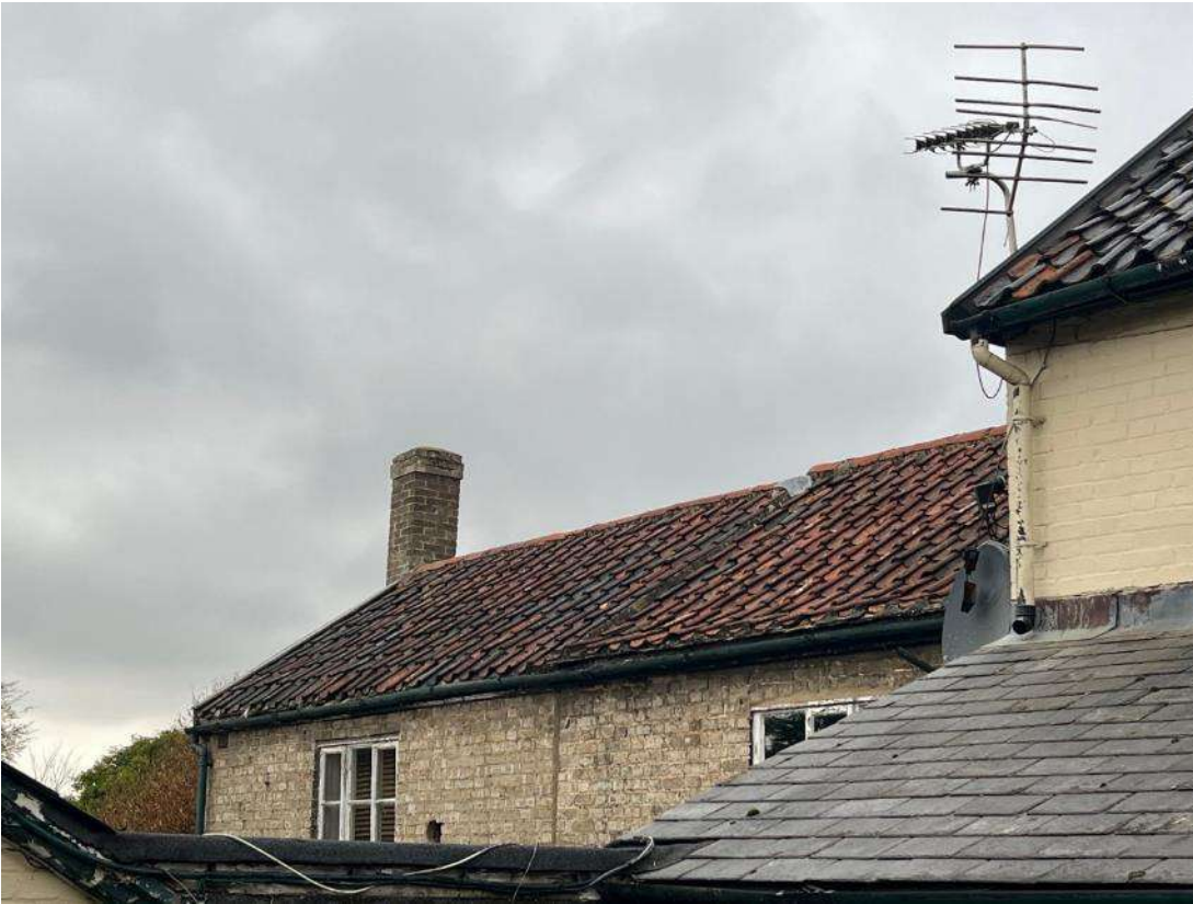
Photo 15. Building 3 (ref B3A). East aspect of building.
