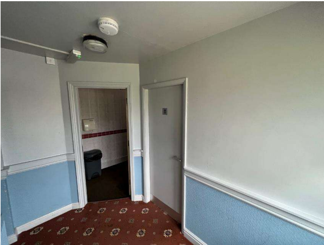
Photo 4. Internal view of building 1. Lobby to toilets.
