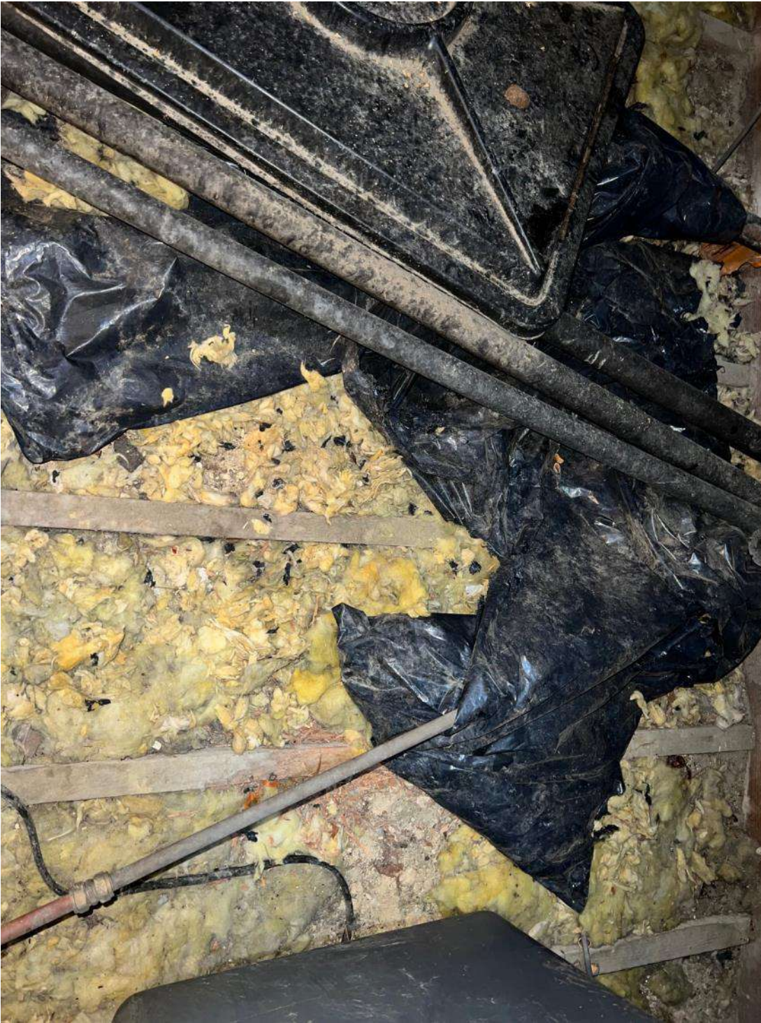
Photo 14. Building 2 (ref B2A). Likely evidence of squirrel damage. A squirrel has been seen to enter the roof space of building 3 on multiple occasions during the survey visits.
