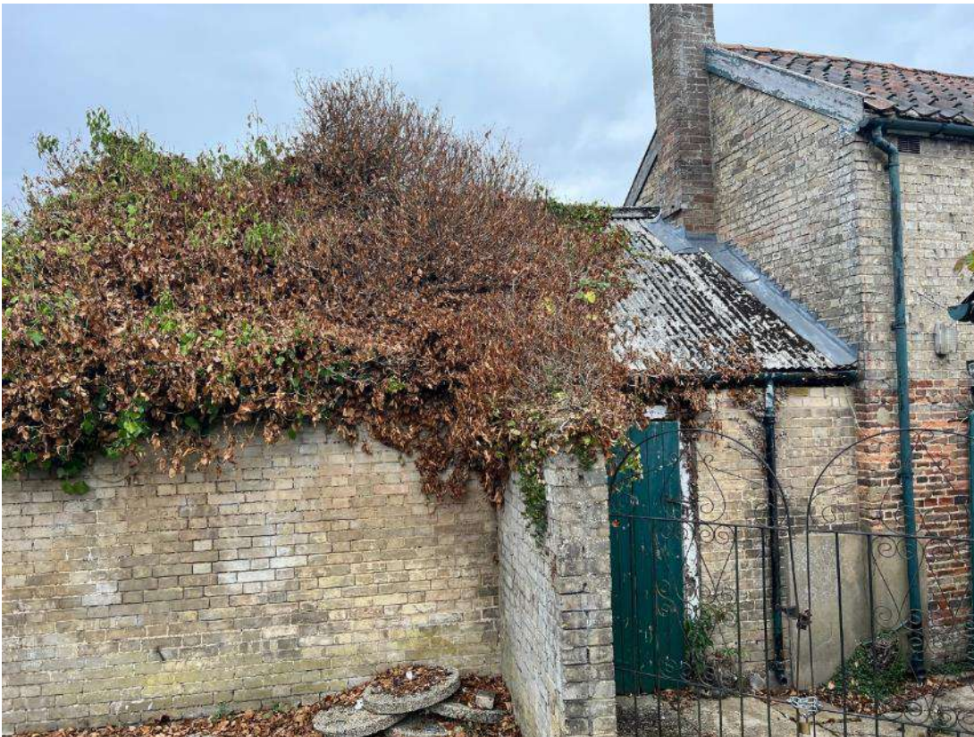
Photo 22. Building 4 (ref B4). Shows building 4 built up to building B3A. Most of the roof is covered in dense ivy growth.
