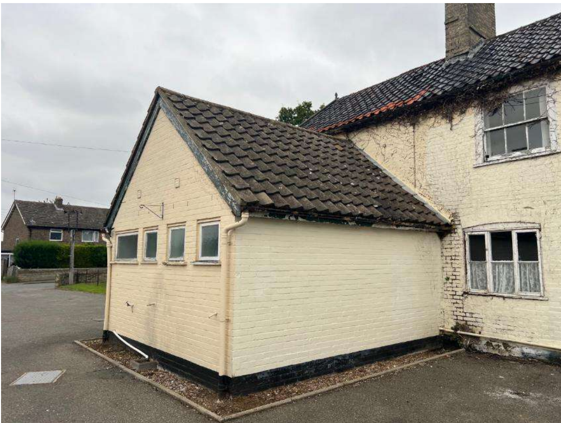
Photo 2. Building 1. Rear of building, adjoining to building 2 (ref B2A).
