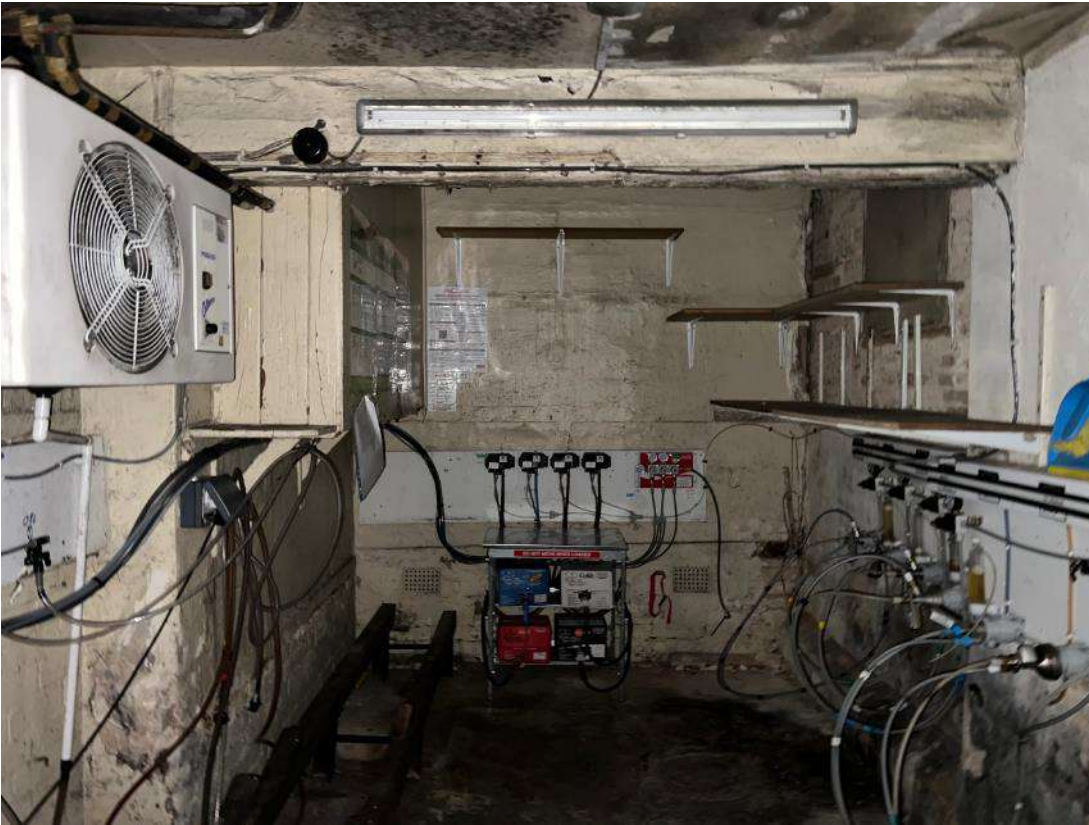
Photo 31. Cellar at base of building 3. Looking south.
