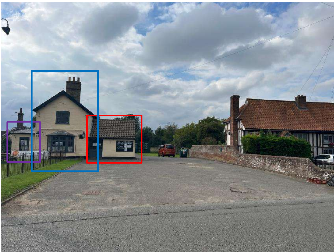
Photo 36. Taken from the road, looking at extensive area of tarmac, providing access and parking for the tavern. Grassland area 1 along with metal railings are also shown. Building 1 is shown in red, building B2A is shown in blue and building B2B is shown in purple.
