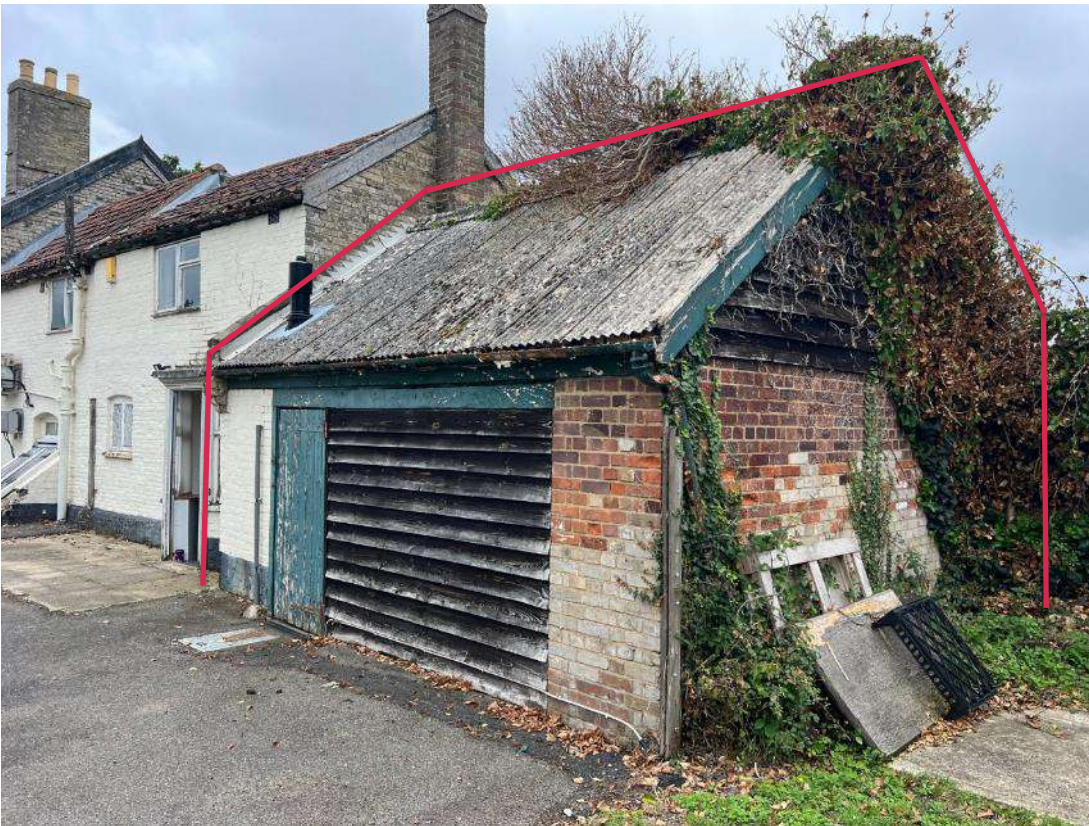
Photo 21. Building 4 (ref B4). Outline of building shown in red. Shows western access point and timber cladding. There is a corrugated cement roof.
