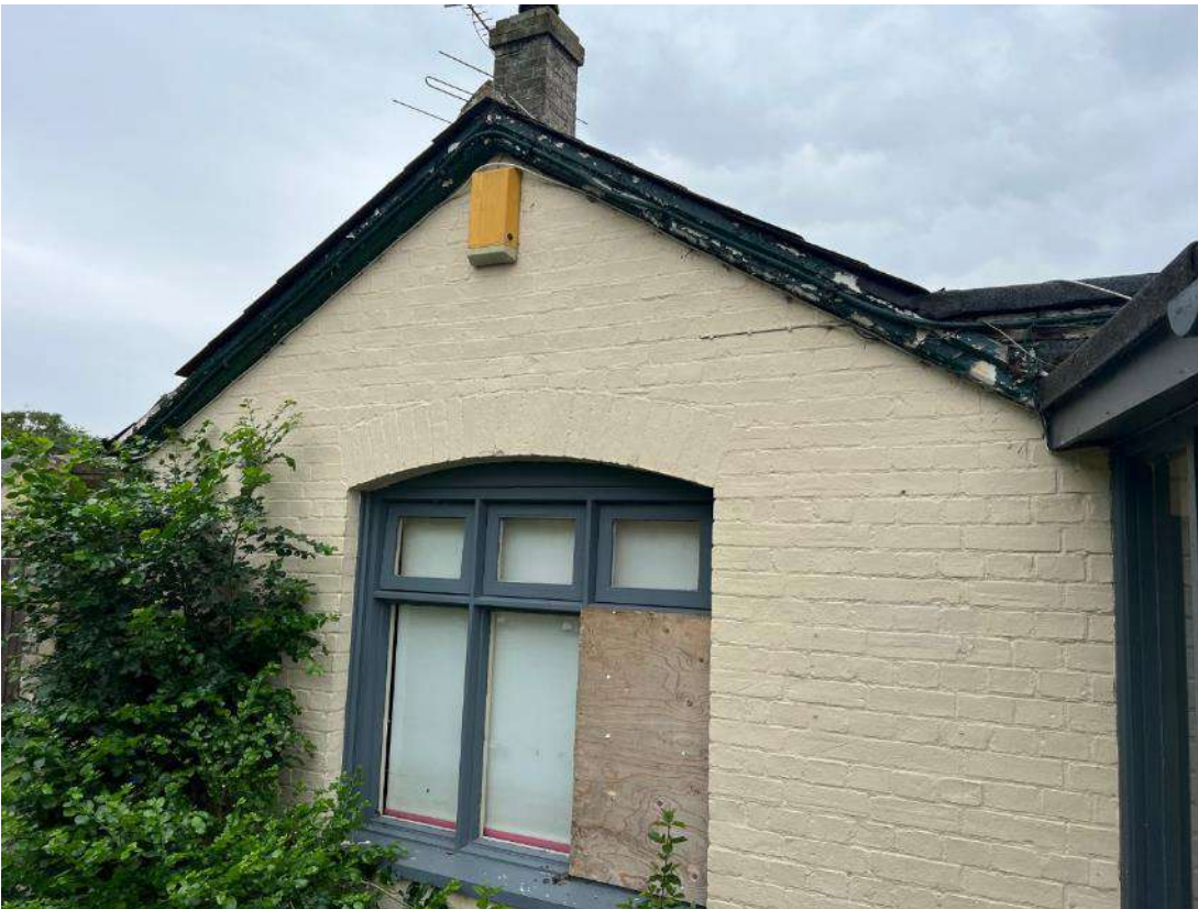
Photo 28. Building 5. Shows northern gable end.
