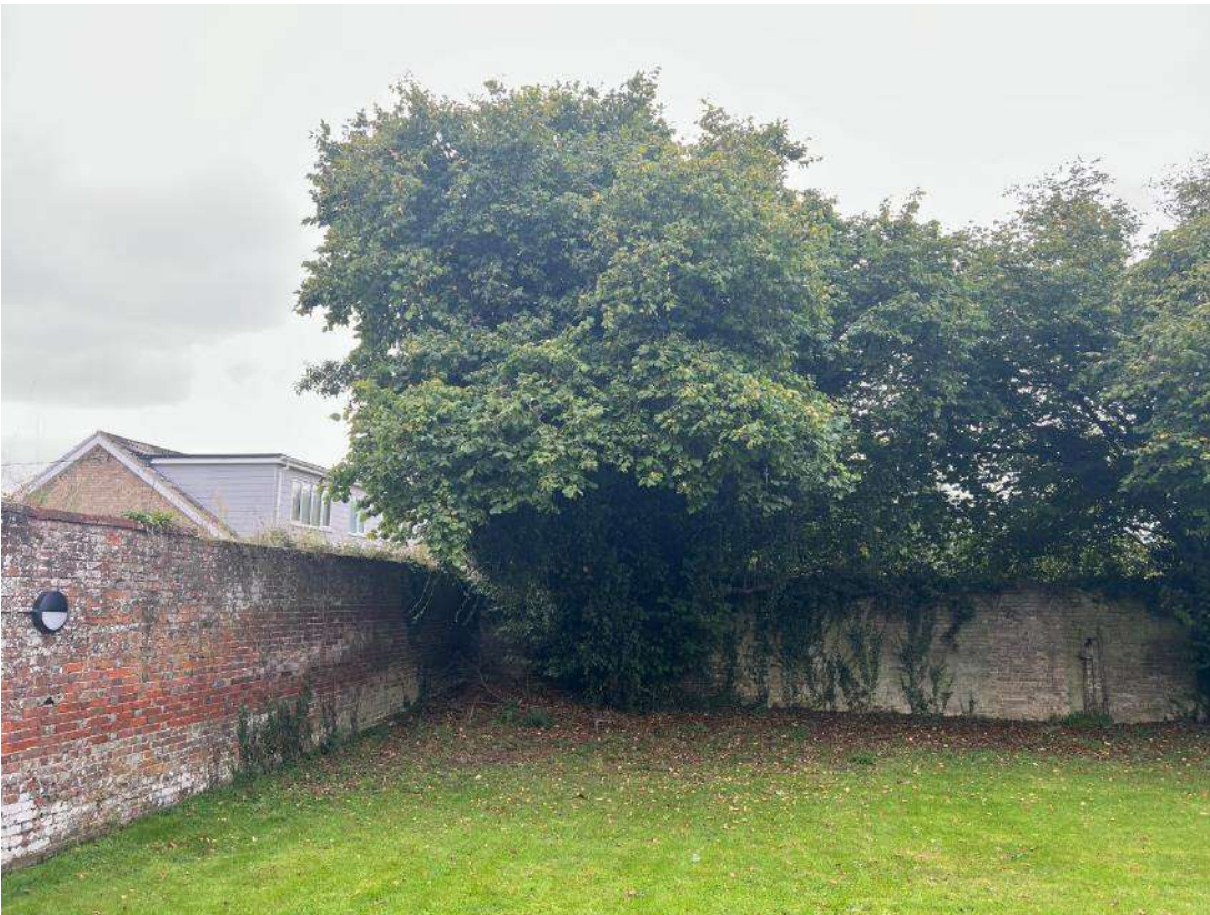
Photo 42. Shows south eastern corner, where ancient hazel stool (T1) exists alongside brick wall boundary. Also shows short grass sward in grassland area 3.
