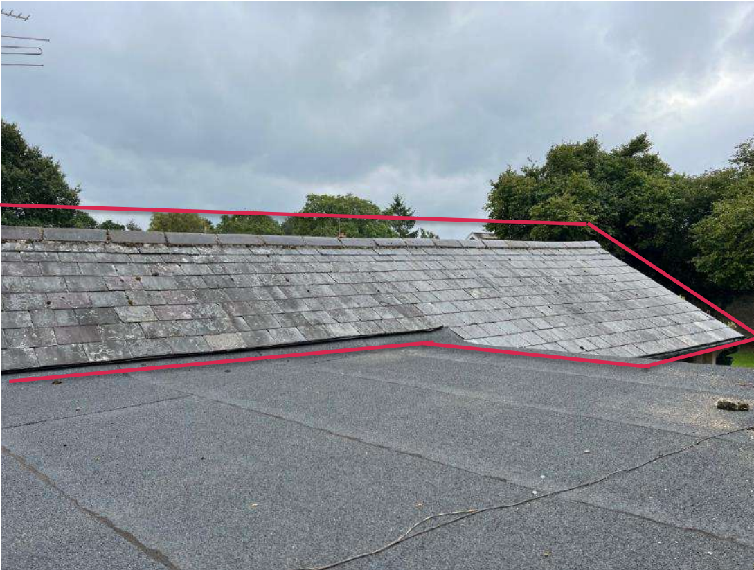
Photo 29. Building 3 and building 5. Shows building 5 slated roof as outlined in red.
