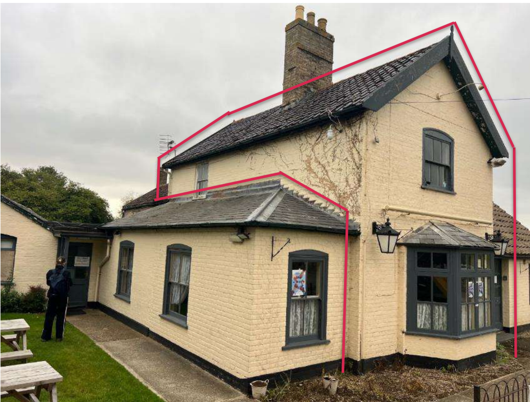
Photo 11. Building 2 (ref B2A and B2B). Building B2A is outlined in red.
