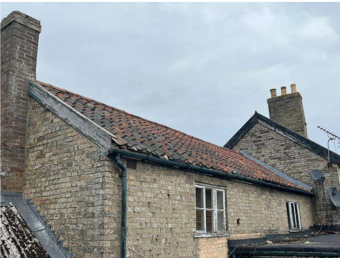
Photo 17. Building 3 (ref B3A) adjoining building B2A. East aspect.
