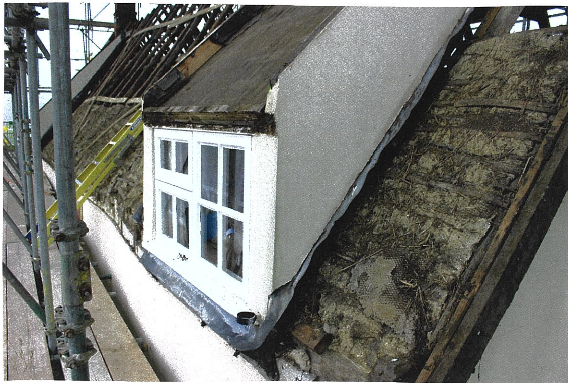
DORMER AFTER ROOF STRIPPED FOR REPAIRS
