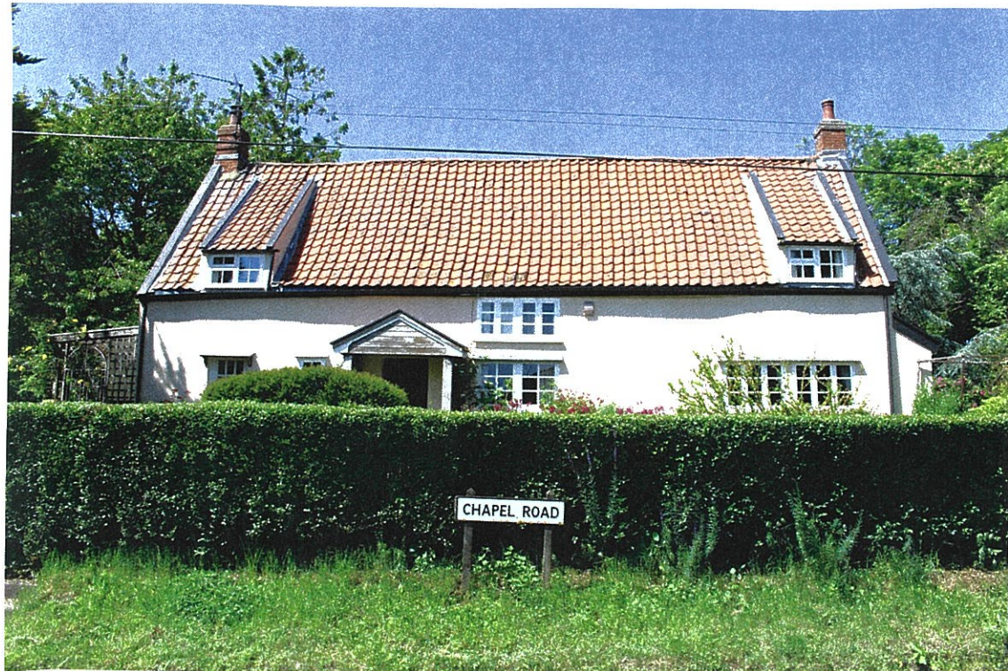
FRONT (SOUTH) ELEVATION TO THE ROAD.
