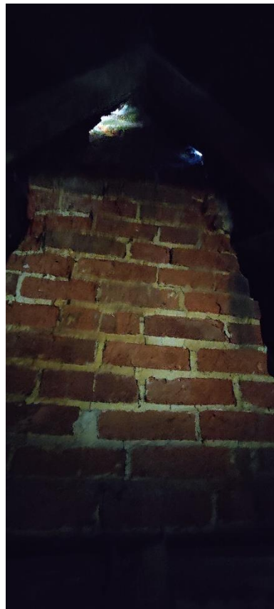
Photo 6 Interior of loft – west chimney stack showing brick work and light gaps at edge of roof
