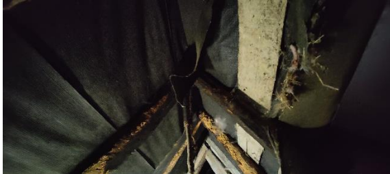
Photo 8 Interior of loft – west end showing felt lining and damaged roof timbers
