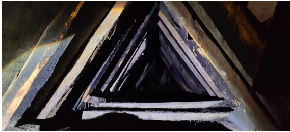
Photo 8 Interior of loft – west end showing felt lining and damaged roof timbers
