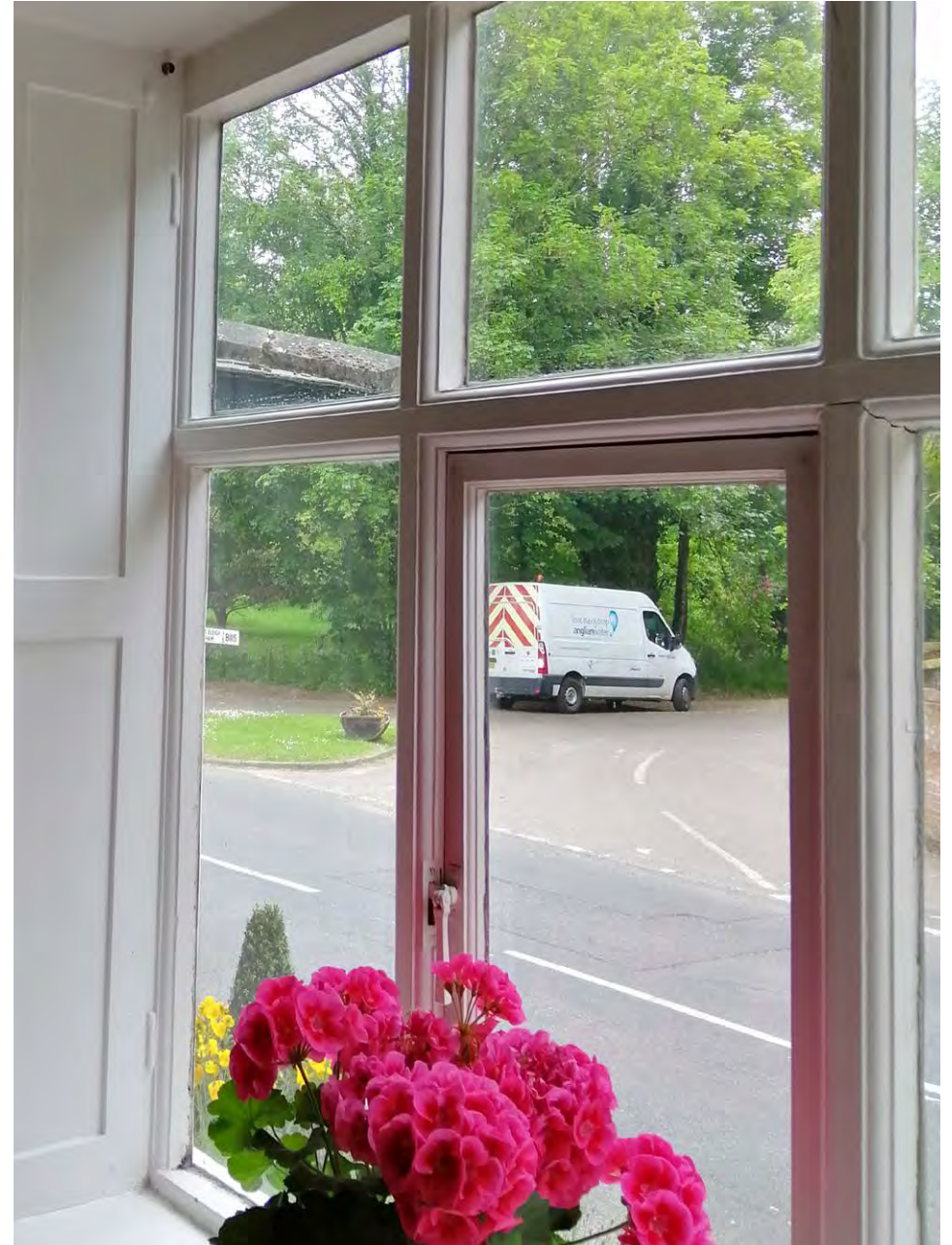
19th Century window WG02 on ground floor in the drawing room, which is to be retained without alteration. The frame and casement profiles for the proposed replacement windows in this area of the house are based primarily on this window.
