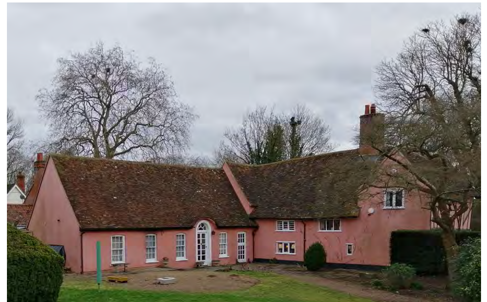
Jackdaws Ford viewed from the northwest, showing the northern wing (left side) and the northern elevation of the western cross-wing and central hall (right side).
