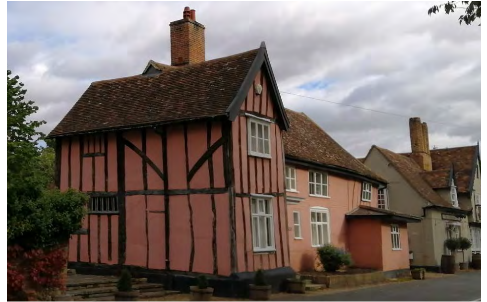
Jackdaws Ford viewed from southwest, showing the original mullion windows (one blocked) on the west elevation and the mixture of 19th and 20th century windows on the south elevation.
