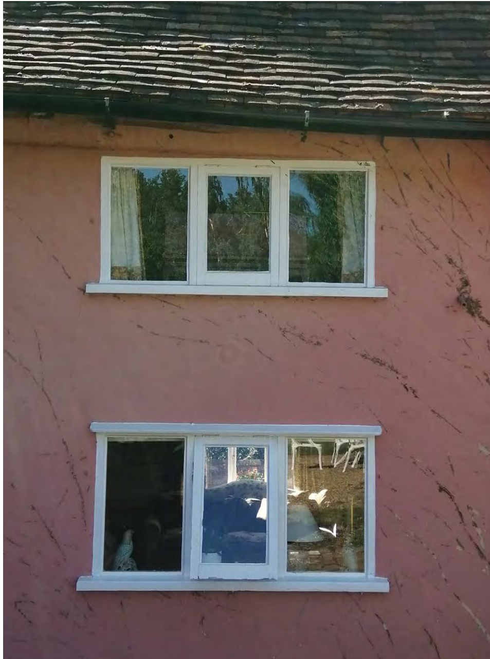
Windows WG07 (below) and WF08 (above) viewed from the exterior (both to be replaced).
