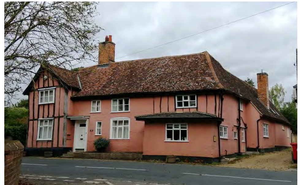
Jackdaws Ford in 2023 viewed from the southeast. Two windows (in the area of the front door) have been added, the door to the former butcher's shop has been removed, and the ground floor window in the western crosswing has been replaced since the 1870 photo above.. (Image published online at Chelsworth.org.uk)
