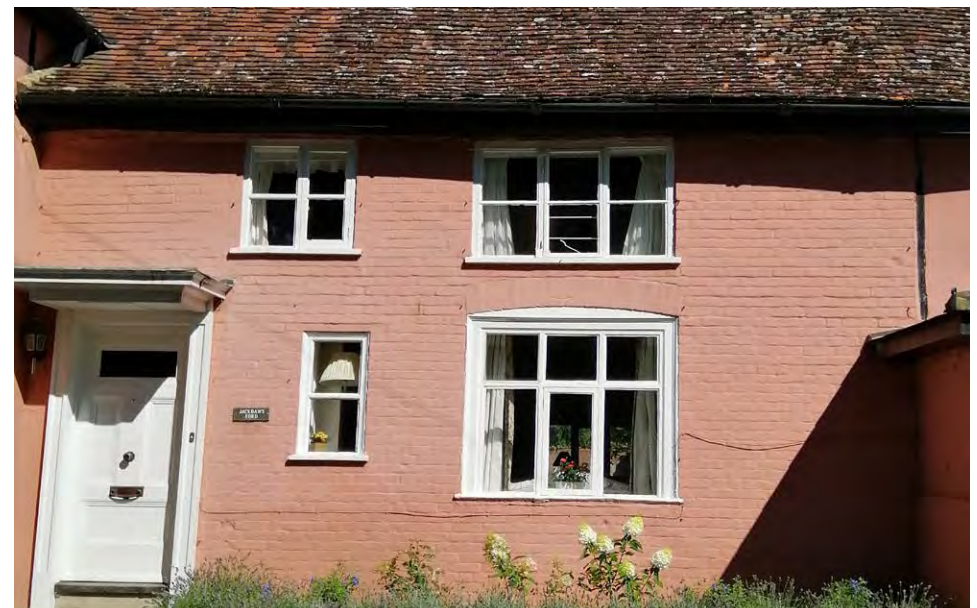
Jackdaws Ford viewed from the south. The windows on the right hand side are 19th Century windows to be retained, while the two smaller windows on the left hand side are 20th Century windows to be replaced.
