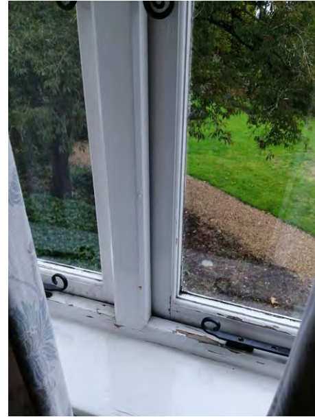
Window WF08 viewed from the interior (to be replaced).
