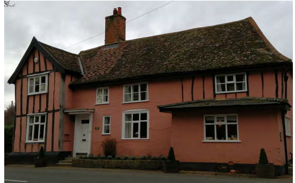
Jackdaws Ford viewed from the southeast, showing windows within solid brick walls in the central hall area and in the former butcher's shop extension (RHS)
