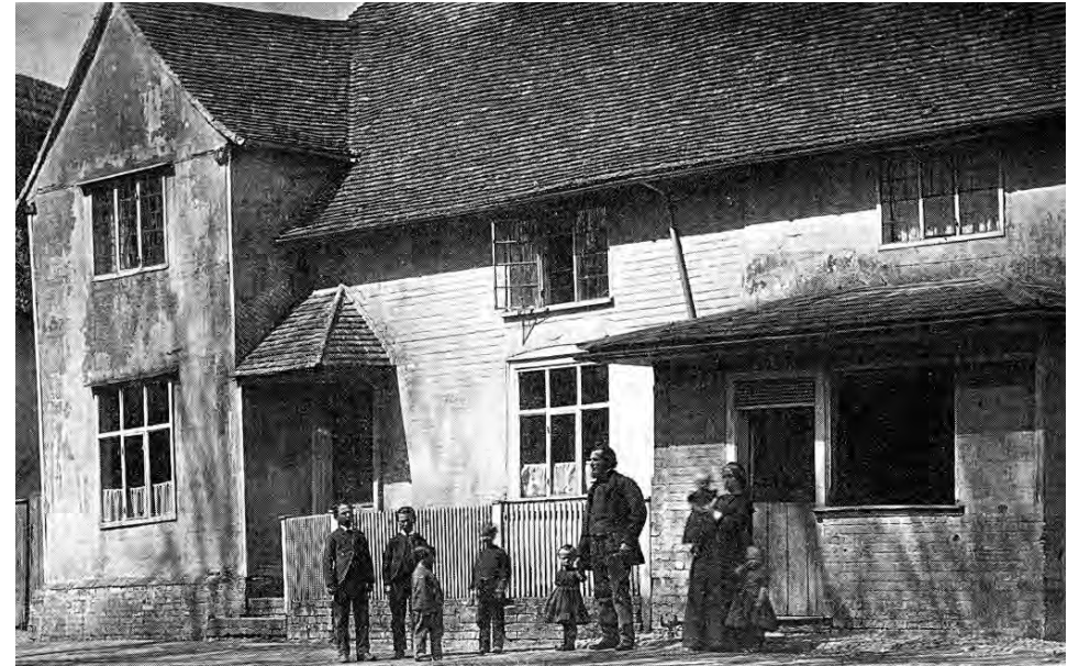
Jackdaws Ford in 1870. The 3no. first floor windows and the centre window on the ground floor remain, though the casements have been replaced since this photo. (Image published online at Chelsworth.org.uk)
