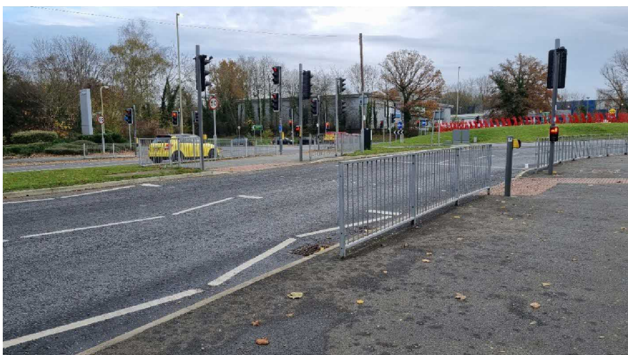
Photo 23: Signalised crossing facilities at southern end of Crockford Lane
