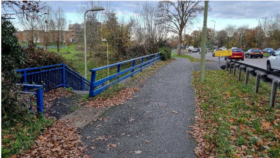
Photo 29: Looking north toward parapet adjacent to A33
