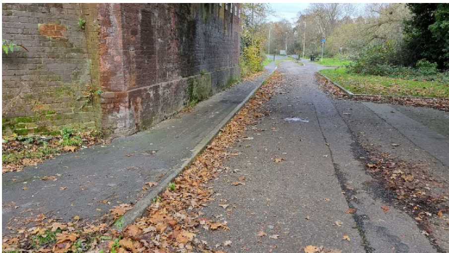
Photo 25: Route on disused road beneath railway line
