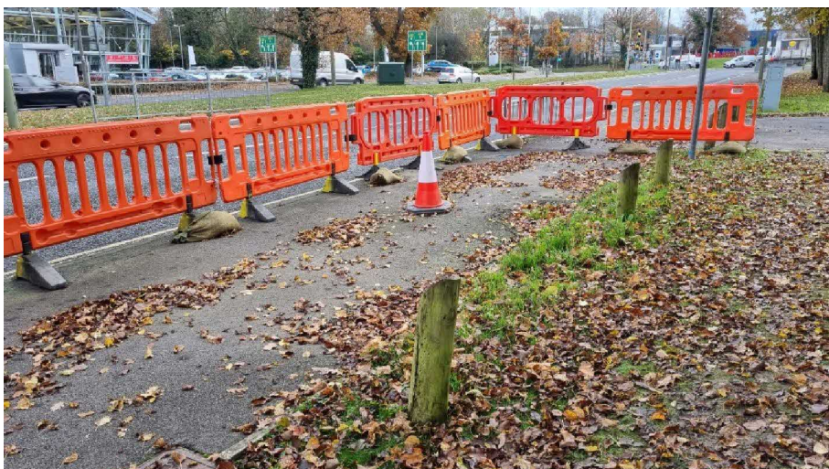
Photo 21: Temporary closure of Crockford Lane western footway / cycleway
