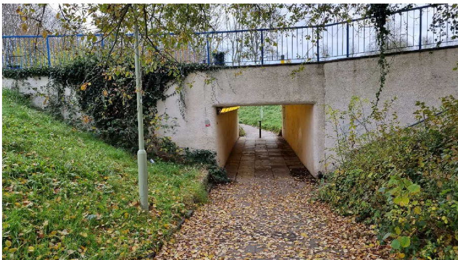
Photo 27: Looking south towards underpass beneath Carpenters Down
