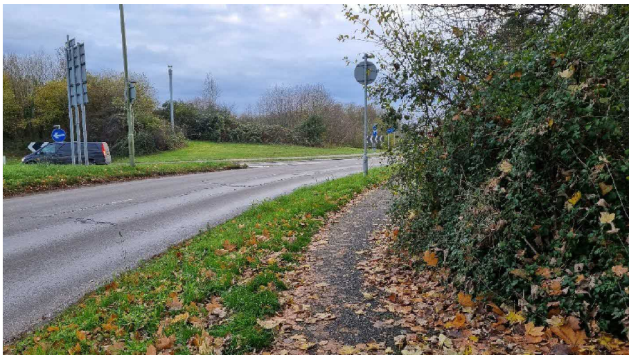
Photo 30: Looking north towards A33 / A339 roundabout
