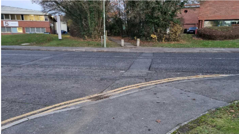
Photo 14: Looking east towards crossing point on Lime Tree Way
