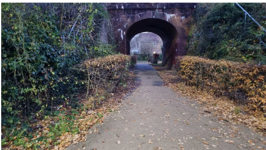
Photo 16: Looking east towards bridge passing beneath railway
