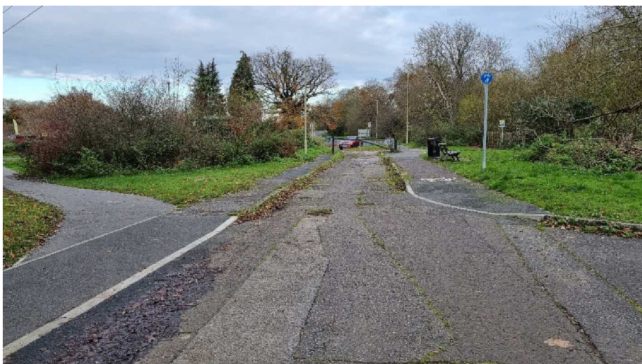
Photo 26: Eastern end of route on disused road, looking east
