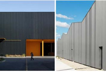
The principal cladding across the scheme is a profiled metal cladding. The profile is to be laid vertically with a small sinusoidal (rounded) profile. The material provides an industrial aesthetic and visually emphasises the form of the building and roof pitches.
