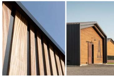
Timber cladding is used to contrast the dark metal profiled cladding. Timber provides a material that is visually warmer and compliments the strong lines of the cladding.
