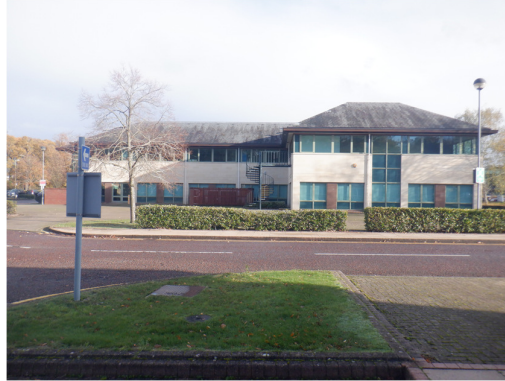
2. Rear of commercial Building 1, viewed from the west.
