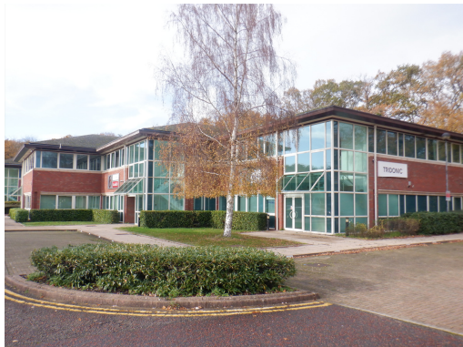
11. Front of the attached northeast buildings (Buildings 5, 6 & 7), viewed from the southeast.
