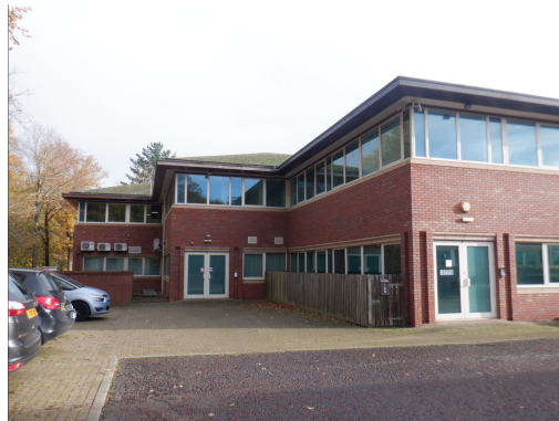
12. Rear of the attached northeast buildings (Buildings 5, 6 & 7), viewed from the west.
