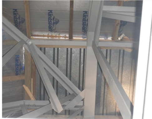
10. Hipped section of Building 1 lined with foil-covered insulation boards.
