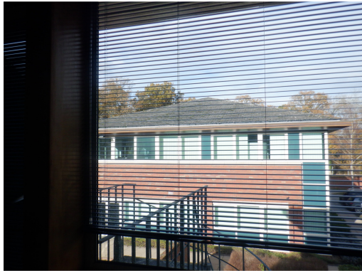
13. Flat slate roof tiles sealed to the roof on Building 4, viewed from the east.
