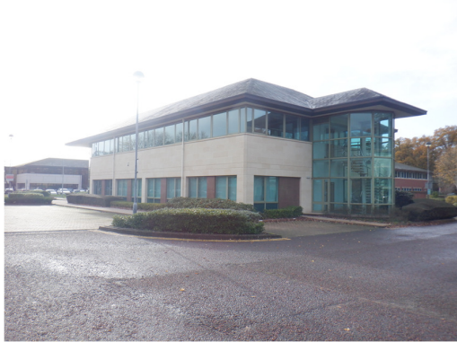
1. Front of commercial Building 1, viewed from the northeast.
