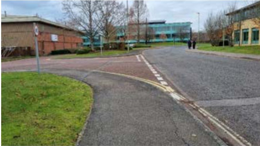
Photo 10: Stag Oak Lane looking west towards Cherrywood access
