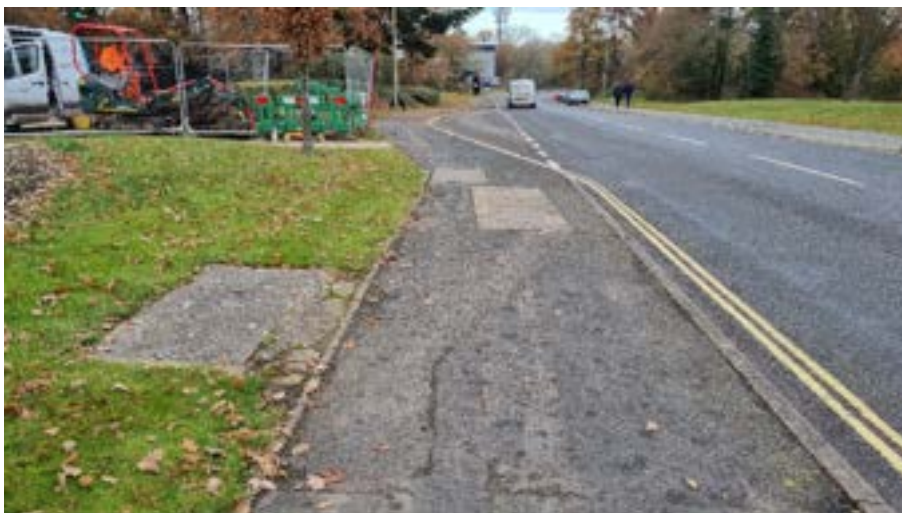
Photo 1: Crockford Lane looking north (at development site frontage)
