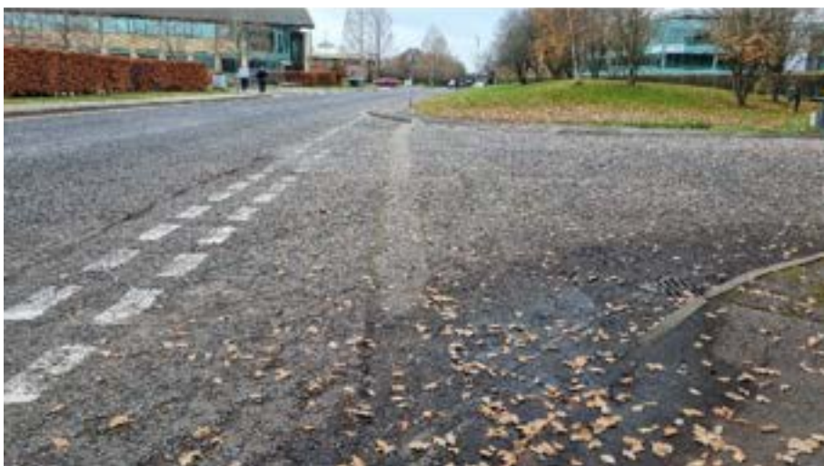
Photo 9: Lime Tree Way, looking south towards Redwood 2 access
