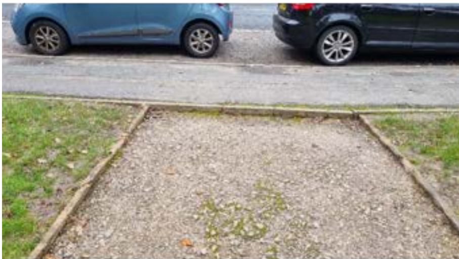
Photo 8: Level difference between path and adjacent footway
