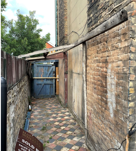
Side Passage to 10 Carson Road
