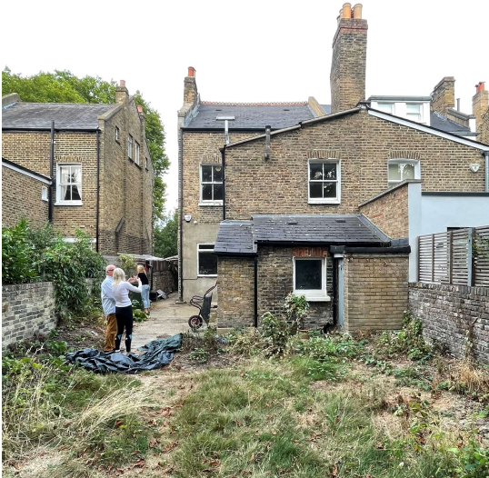
Rear Elevation of 10 Carson Road
