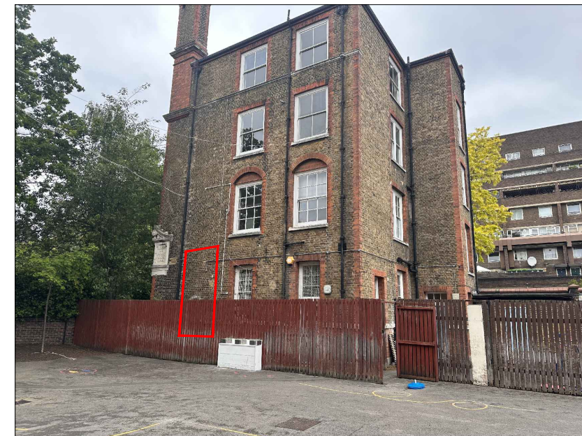
Wall Mounted ASHP Location
