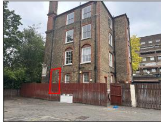
Wall Mounted ASHP Location
