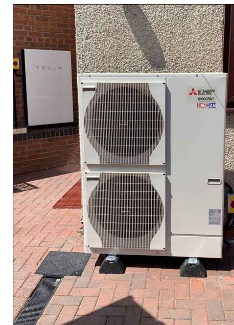
Typical Wall Mounted ASHP
