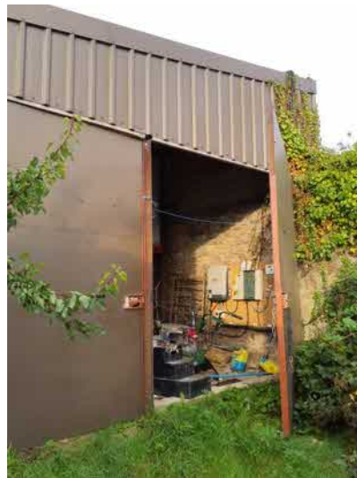
Plate 4: Eastern elevation showing no suitable features for bats
