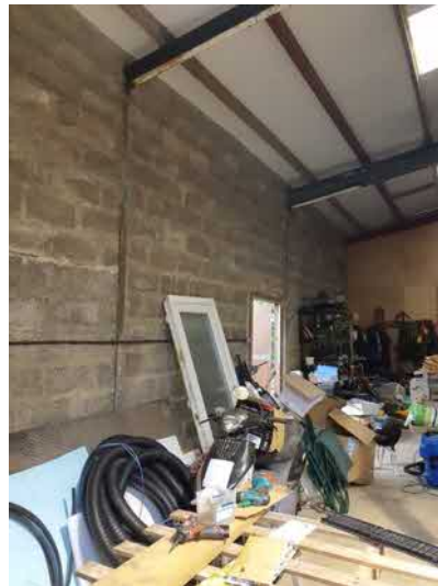
Plate 2: Internal view of barn
