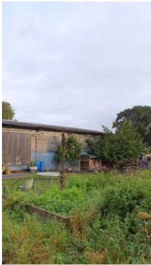
Plate 1: External view of southern elevation showing the corrugated metal roof
