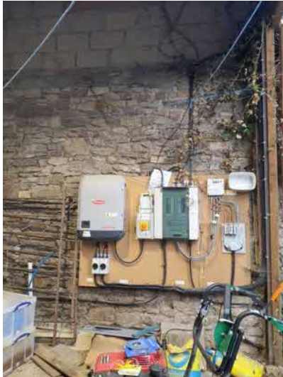
Plate 5: Northern elevation stone wall in good repair with no suitable features for bats
