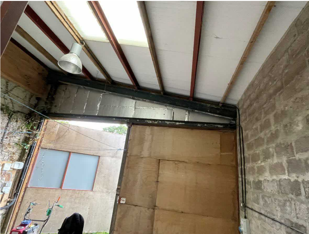
Photo 2 Inside View of the structure along the gable
