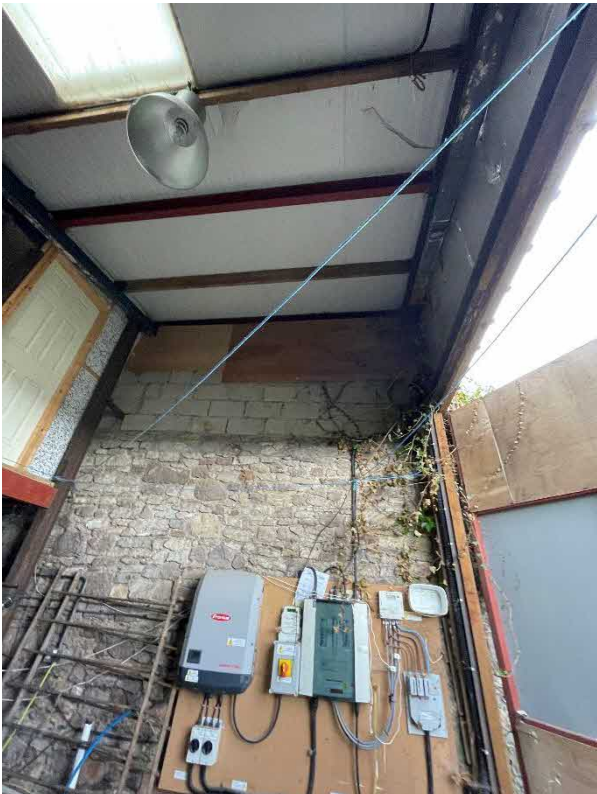
Photo 4 Part view of rear wall
