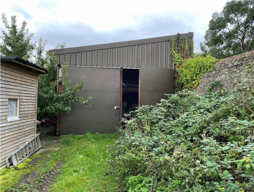
Photo 1 Gable end View of the Barn from the right-hand side
