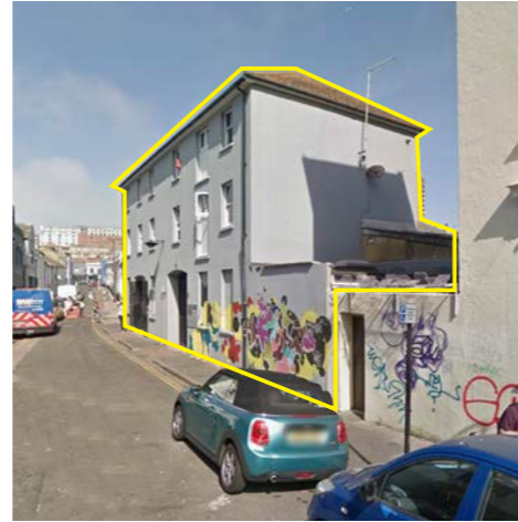
Site Photograph Looking West Yellow outline denotes site envelope
