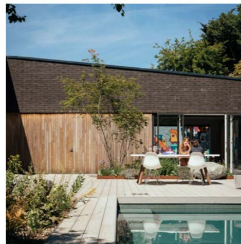
09 New house in Dyke Road, Hove
