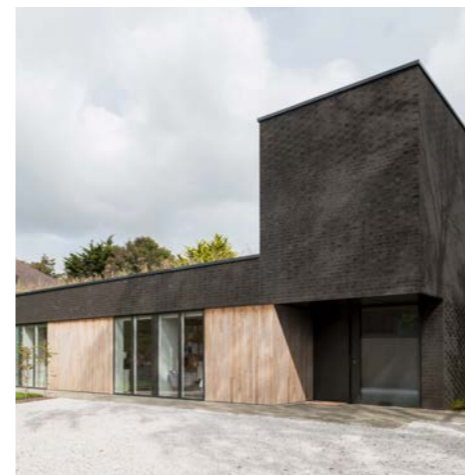
10 New house in Dyke Road, Hove
