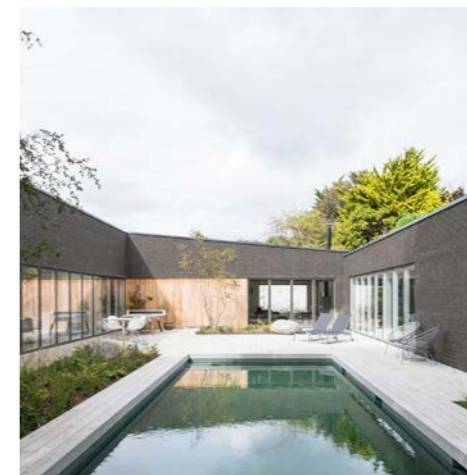
11 New house in Dyke Road, Hove
