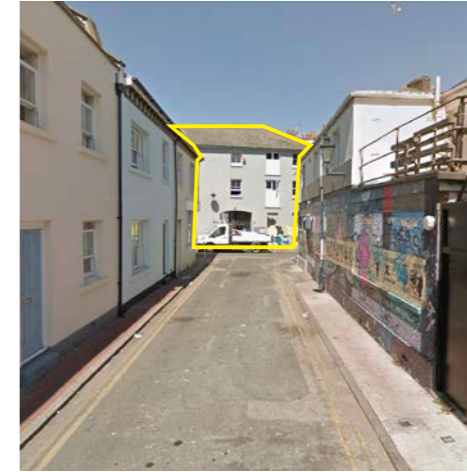
Site Photograph Looking North Yellow outline denotes site envelope
