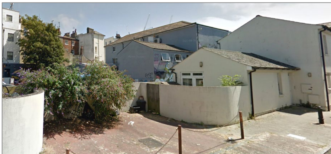
Above: Public street-level view to southeast-west of existing rear of application building. (© Google).
