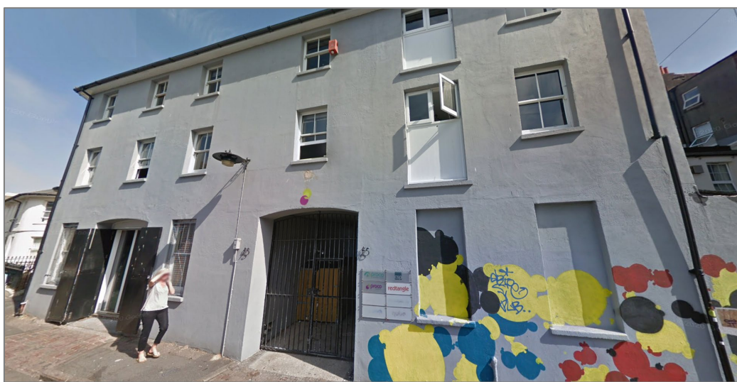
Above: Detail of street-level view of principal elevation of application building. (© Google).
