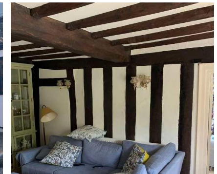
View of Surviving Timber-Framed Structure
