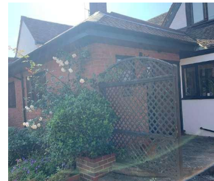
Later Addition to North Elevation
