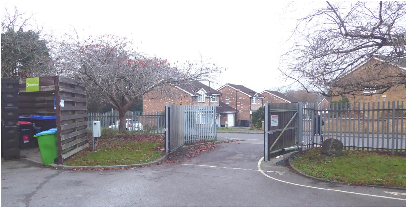
4.4.2 View north west to entrance. Note electrical junction box for existing gates on left by bin store.
