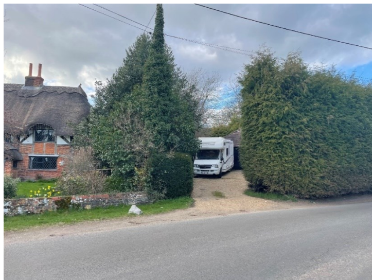
IMAGE 07: Existing Entrance to Tudor Thatch
