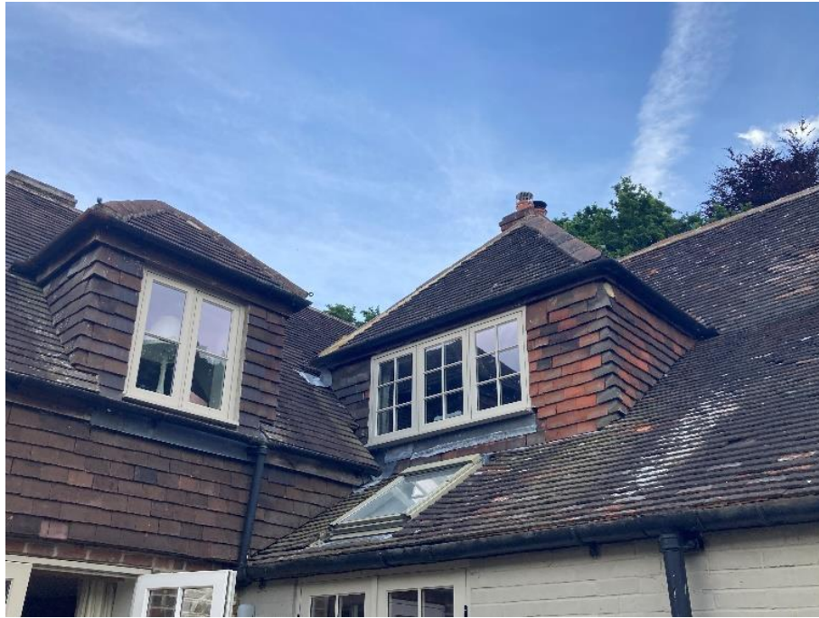
Photograph 3: Hanging tiles present in area which will be impacted
