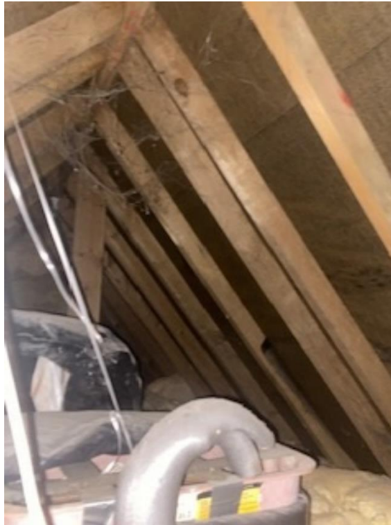
Photograph 1: Felted loft space within the accessible part of the loft space
