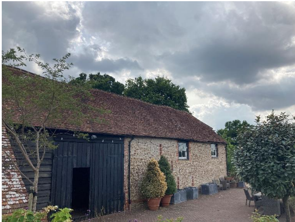
Photograph 5: Single Storey barn with minimal gaps in the tiles
