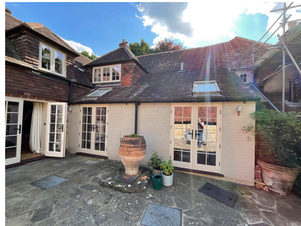
5.3 Photograph of Existing Pitched Roof Dormer
