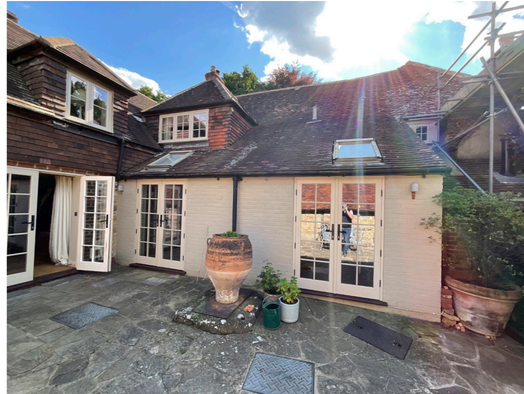
1.2 Photograph of Side Elevation of Main House
