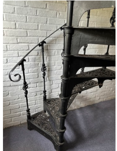
Fig. 4 & 5 Existing spiral staircase, to be removed and replaced with new U-shaped timber staircase within existing aperture.
