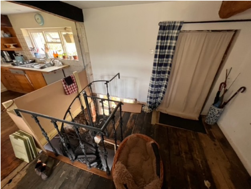
Fig. 4 & 5 Existing spiral staircase, to be removed and replaced with new U-shaped timber staircase within existing aperture.
