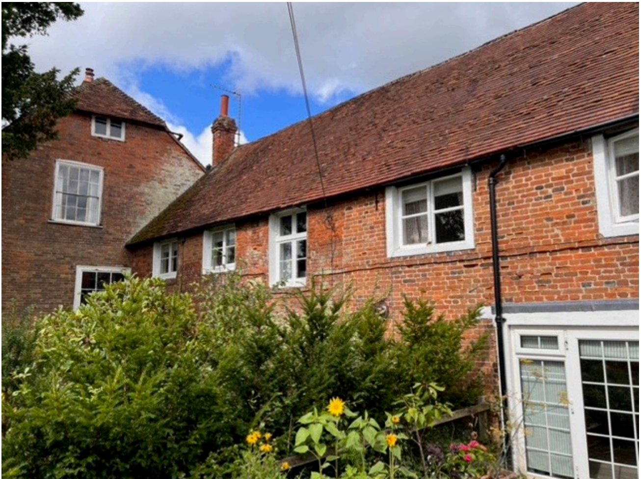
Fig.1. Front Elevation of The Little Malthouse
