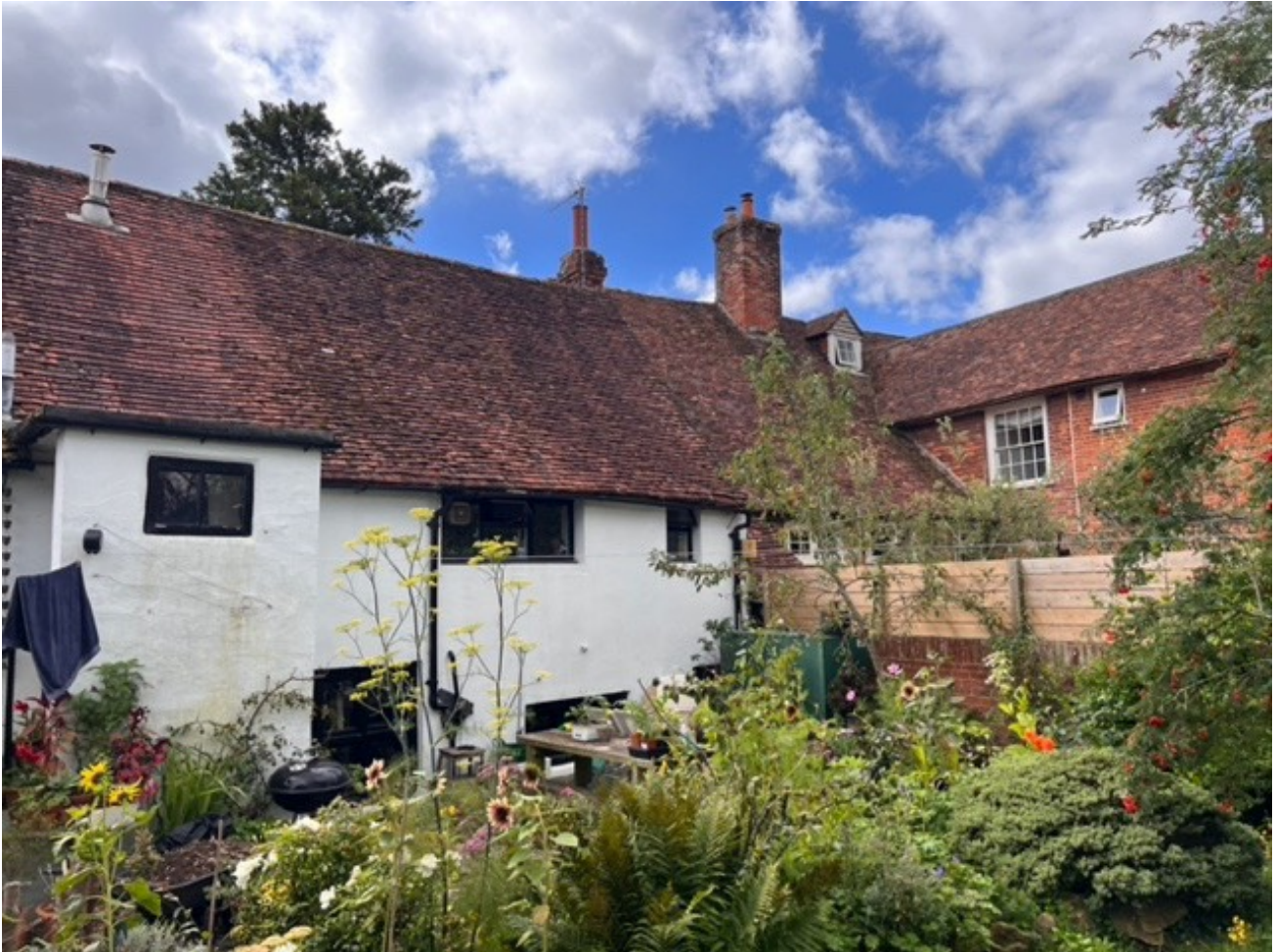
Fig.1. Rear Elevation of The Little Malthouse
