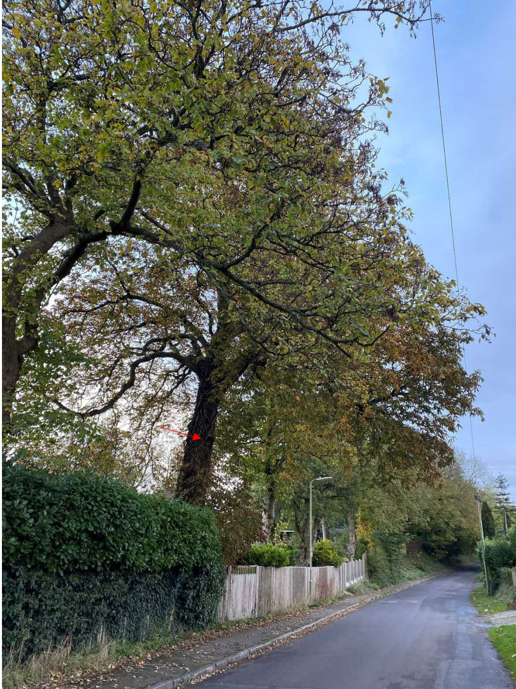
SAL2 T1 horse chestnut (identified by red arrow) with over long branches over the highway. T2 sycamore to the far left of the image.
