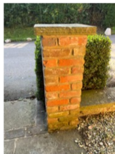
Brick pier, 20th Century brickwork.
