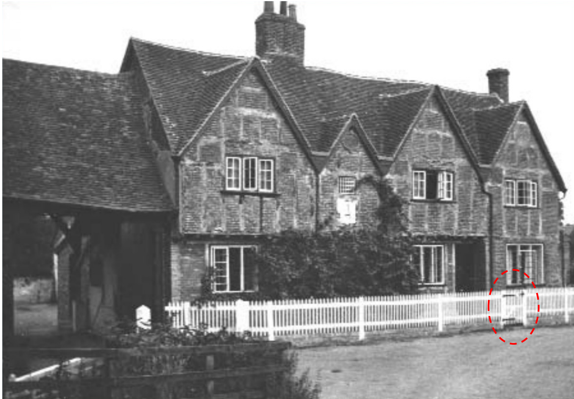
Figure 17: Historic photograph showing Crafton Farmhouse with a picket fence on a low wall, no brick piers and a wooden gate.
