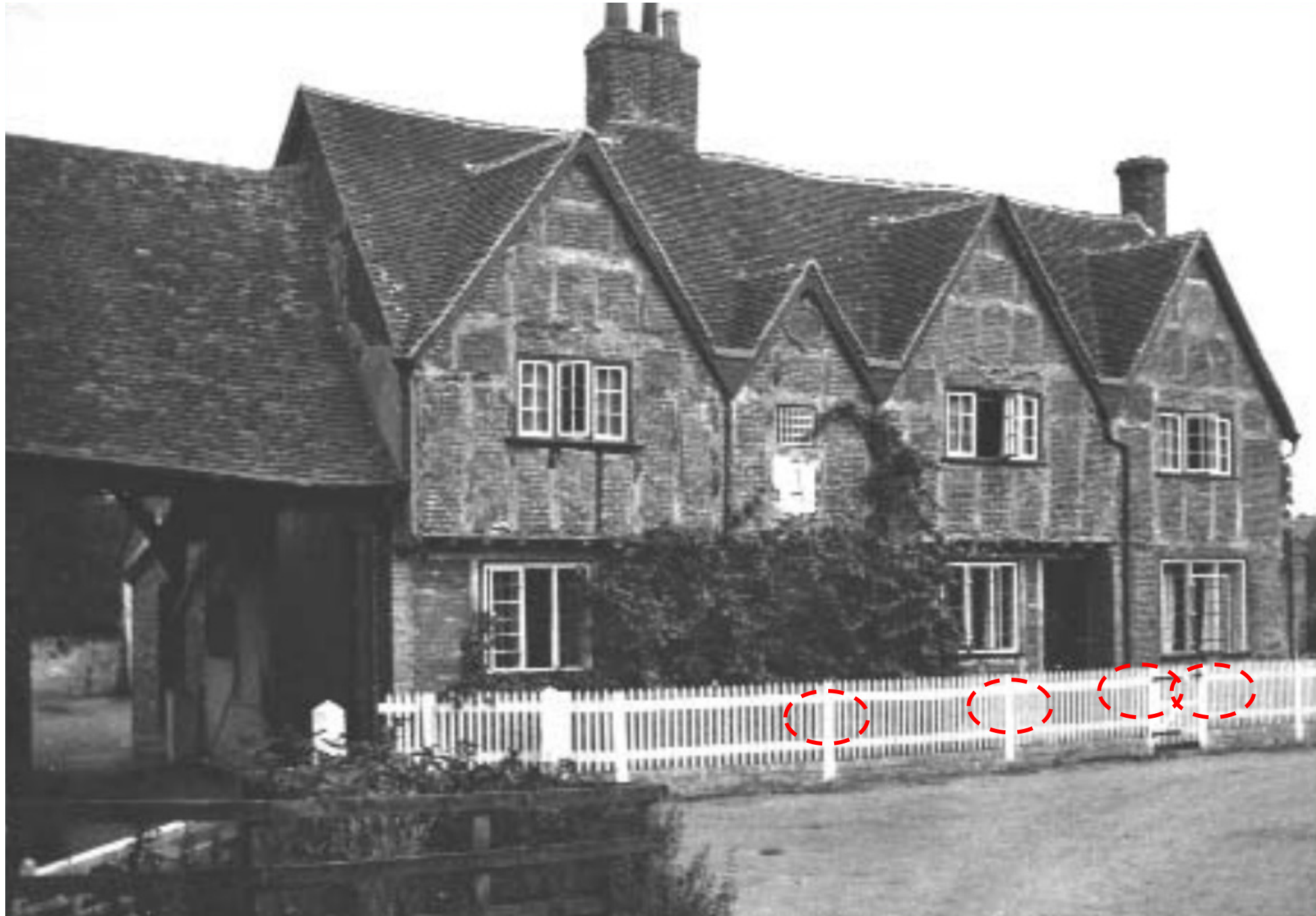
Figure 19: Historic photograph showing Crafton Farmhouse with no brick piers.
