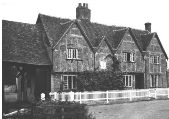
Old image of Crafton Farmhouse with picket fence on low wall with no brick piers.
