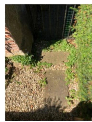
Existing gravel and paving in front of side gate.
