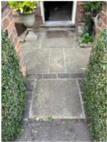
Existing paving seen from road.
