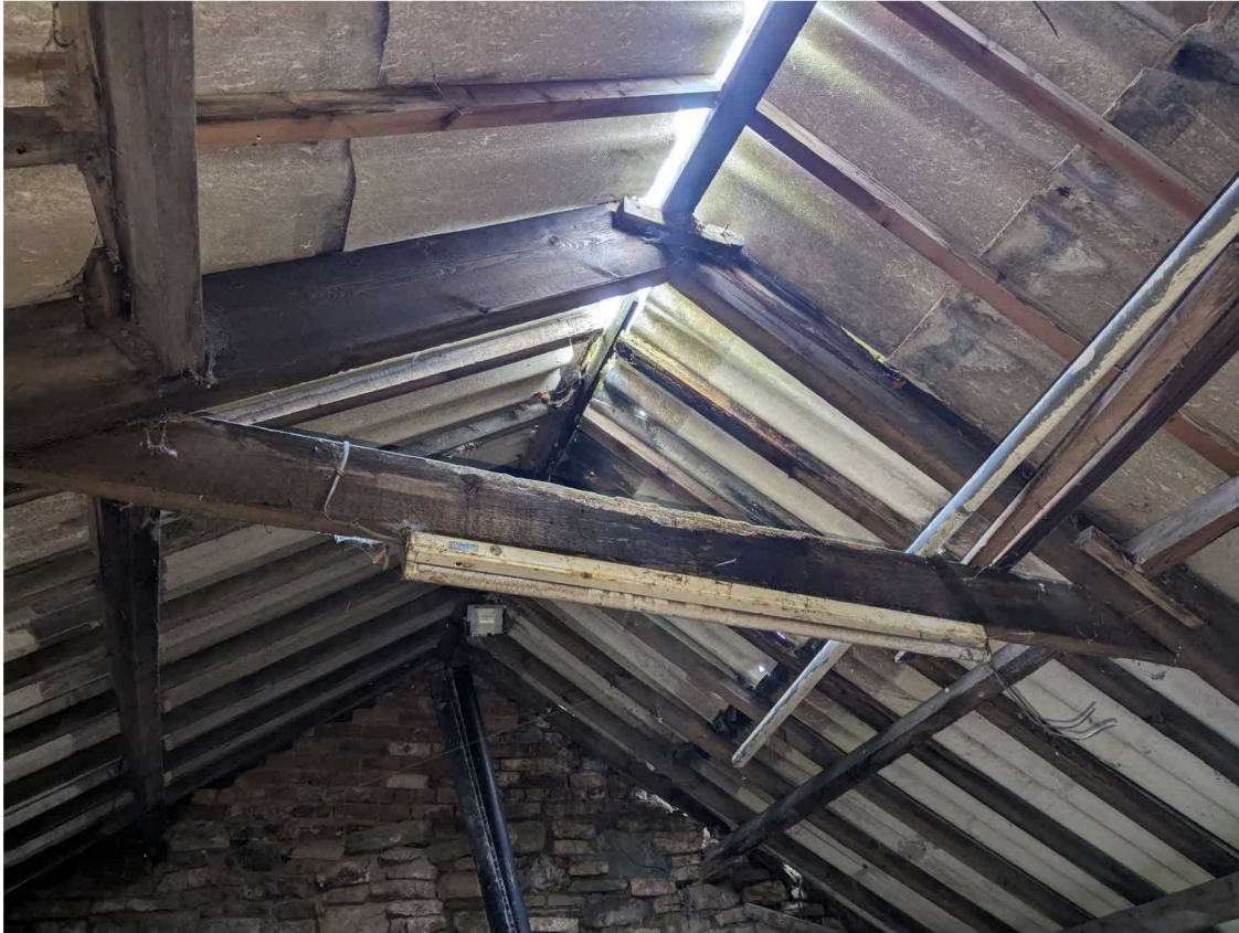
Figure 3 – Existing roof structure
