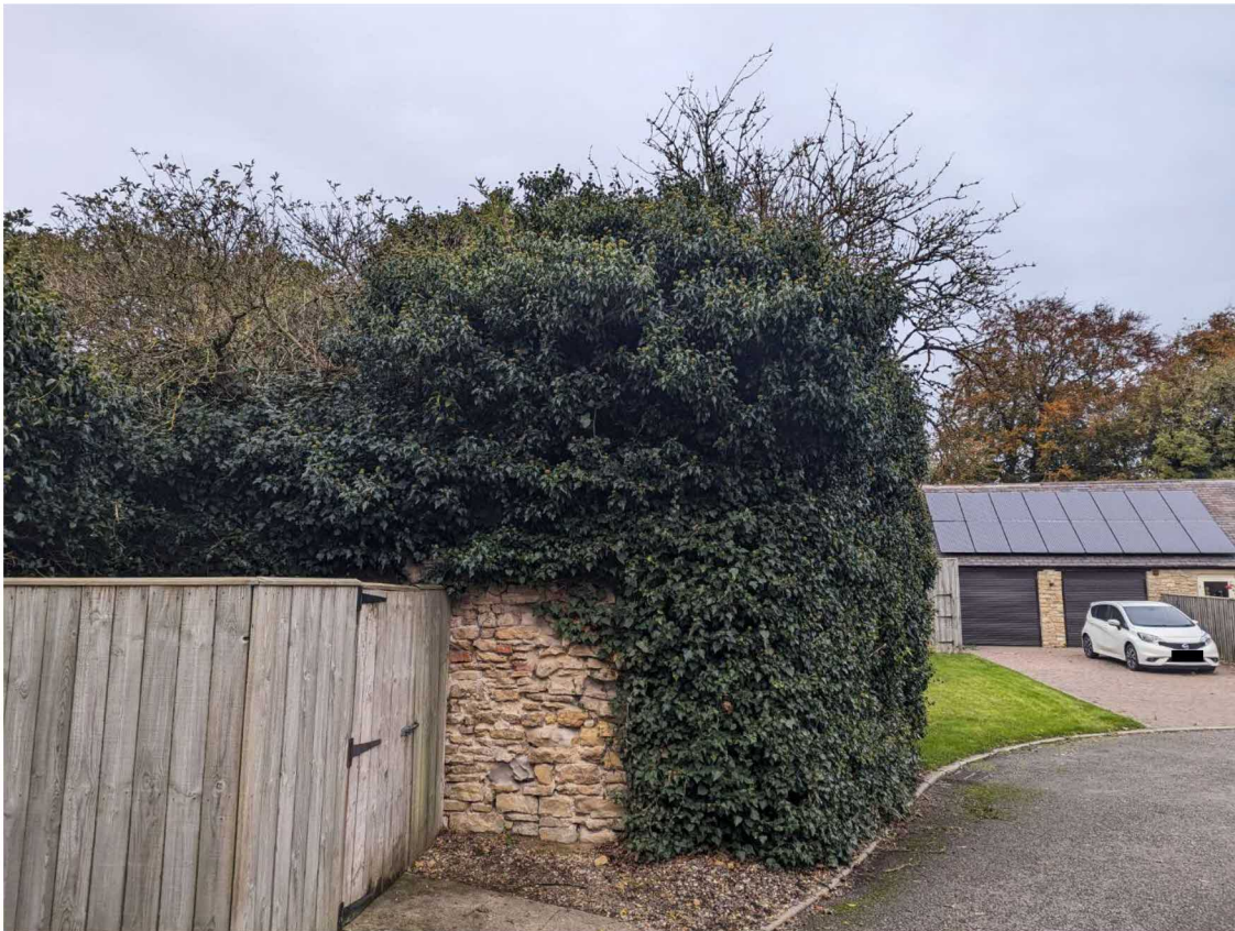
Figure 4 – Vegetation to gable elevation
