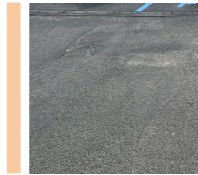
Existing vehicular tarmac to be retained
