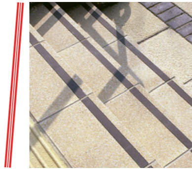
Proposed steps to match paving with Tactile hazard warning Marshalls Perfecta Concrete Step Treads . Risers to match existing brick wall. Colour: Buff Size: 450 x 450mm
