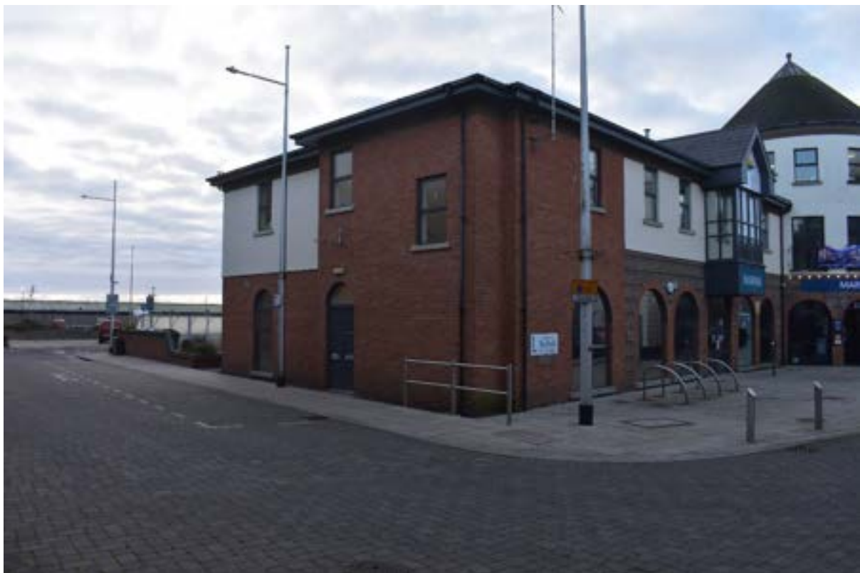
Plate 8: View of the Marina Centre, looking south-east
