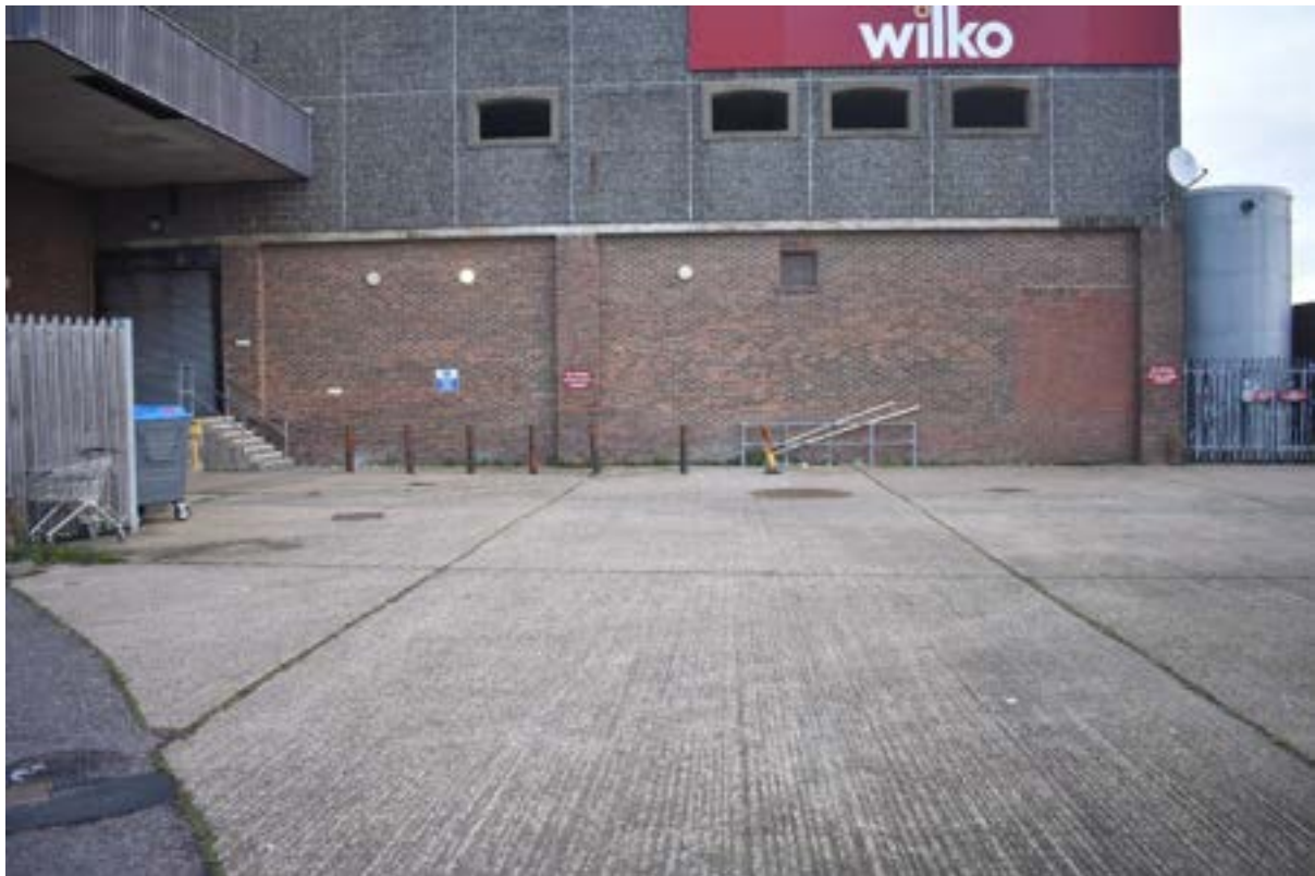
Plate 7: View of the concrete area in the southern corner of the site, looking north-east
