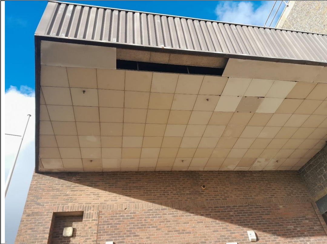
Photograph 3. Potential access points for bats on east face of the Battery Green car park
