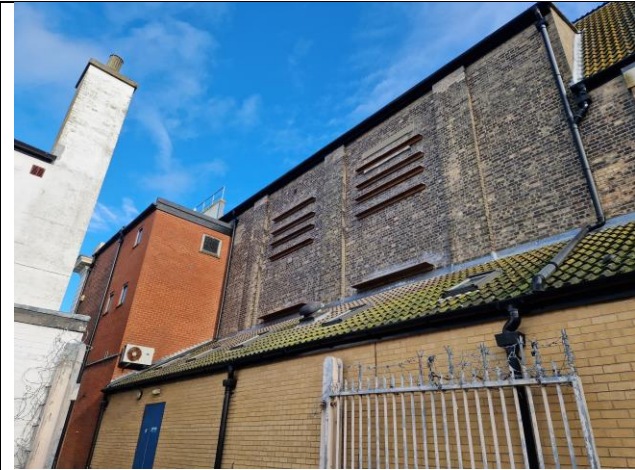
Photograph 5. Kittiwake shelves on western wall of Marina Theatre, provided in mitigation for Eco Lab Avi displacement electric shock system along the main entrance.
