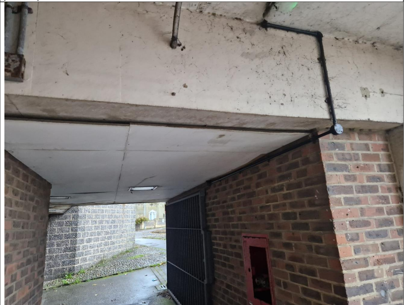
Photograph 2. Carpark walkway ceiling potential bat roost feature
