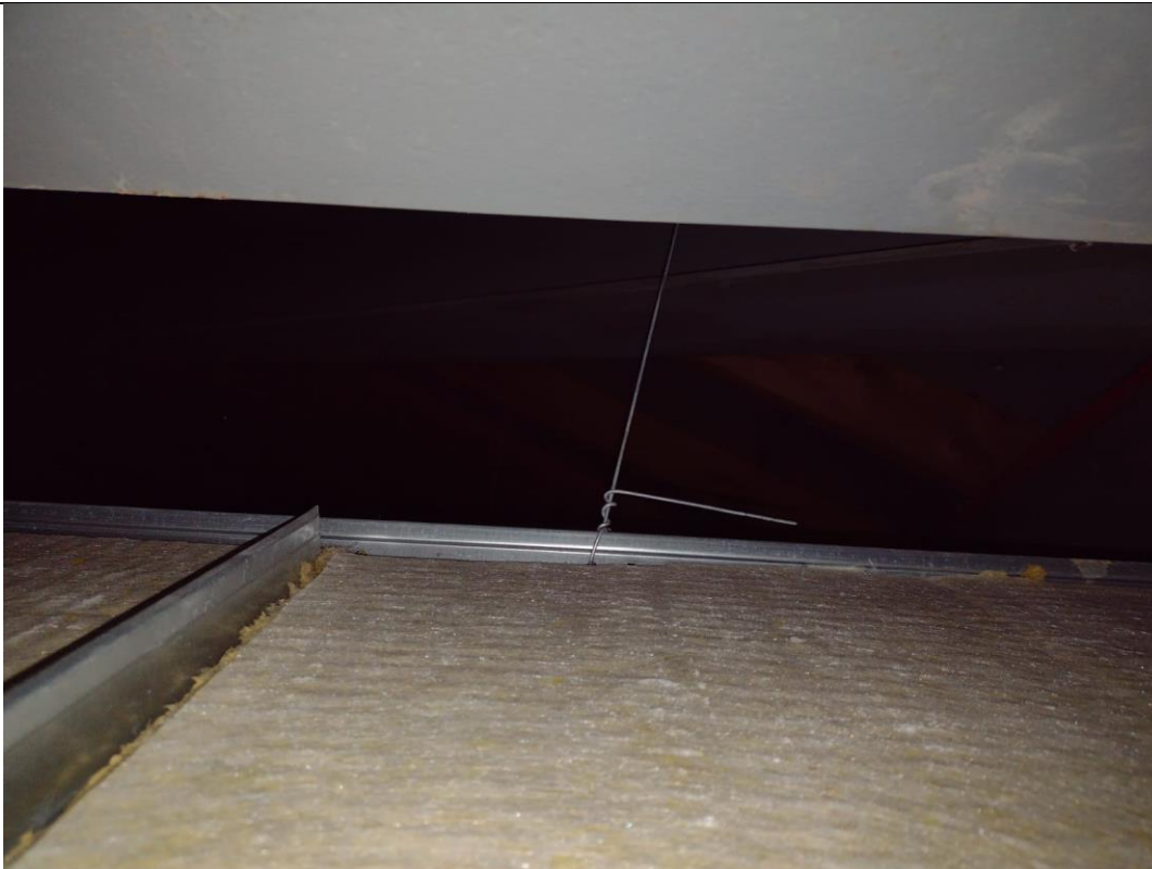
Photograph 4. Internal inspection of roof space of Marina Centre
