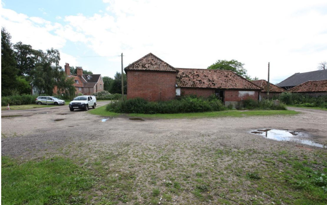
Illus. 3. A general view of the site from the barn (1) to the north showing the L-shaped brick stable flanked on the left by the house (8) and on the right by the uniformly pantiled small brick cart-shed (4) and the open-sided flint-rubble shelter-shed (5). The large building in the rear to the right is a late-20 th century covered cattle yard.
