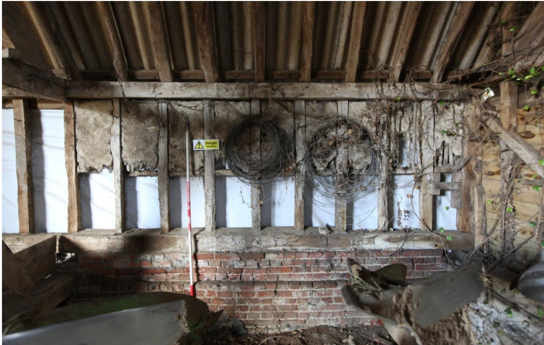
Illus. 13. The back wall of the easternmost bay (1). The narrow studs are tenoned to the roof-plate and sill but only every third stud is pegged. Framing of this kind indicates a date in the 18 th century, as does the uniform brickwork of the tall brick plinth, although the diagonal primary brace in the gable to the right is more consistent with the 19 th – as is the fact that the internal aisle tie-beams are butt-jointed and strapped to the roof-plates. The wattle-and-daub between the studs is an original feature.
