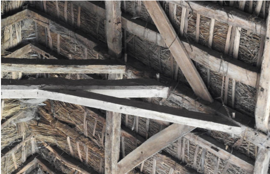
Illus. 7. A detail from the west of the unique central truss of the barn's roof, with double collars and a pair of diagonal soulaces. Trusses of this kind are normally found only in high quality 13 th and 14 th century roofs. Note the step in the principal rafter above the upper collar which indicates it was re-used from a clasped-purlin roof, and the empty mortices in the common rafter to the left which also indicate re-use.
