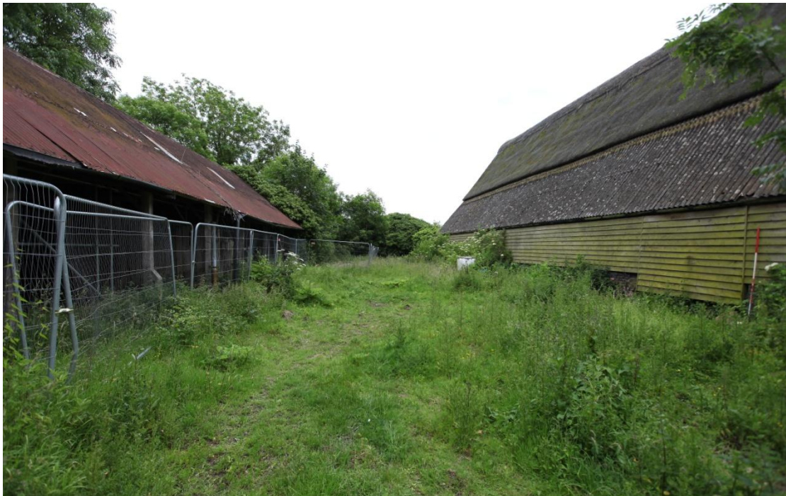
Illus. 4. The narrow yard to the rear (north) of the barn as seen from the west. The long shelter-shed (7) is overgrown and largely inaccessible but the section to the left was largely rebuilt in softwood and corrugated iron during the 20 th century. The barn's rear aisle has been re-roofed in corrugated asbestos and clad in modern softwood but original thatch survives above. The outline of a blocked rear doorway opposite the western entrance is visible to the left of the scale rod with another hidden by vegetation in the rear.
