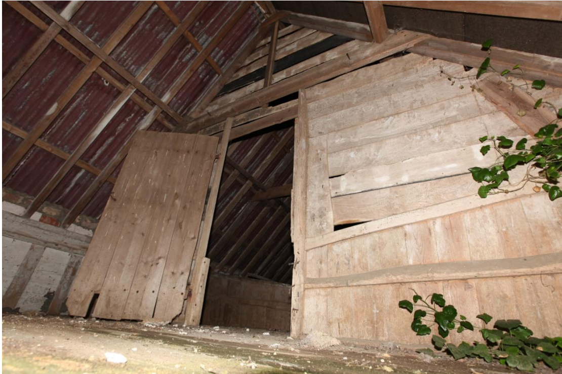
Illus. 21. The cart lodge's loft seen from the north (3) showing a boarded partition with grain bins visible through the door and substantial studs pegged to the roof-plate on the left. The narrow softwood rafters of the clapsed-purlin roof with nailed collars are typical of the mid- to late-19 th century and appear to be replacements. The loft was inaccessible at the time of inspection and this image was taken through the floorboards.
