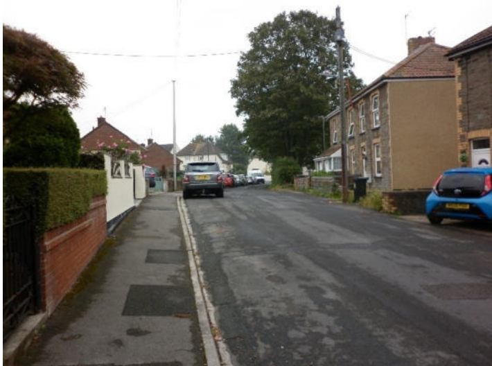
Photo 79: Frys Hill (Facing north by 15 Frys Hill)
