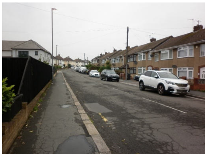
Photo 127: Pound Road (Facing north west by Highview Road Junction)
