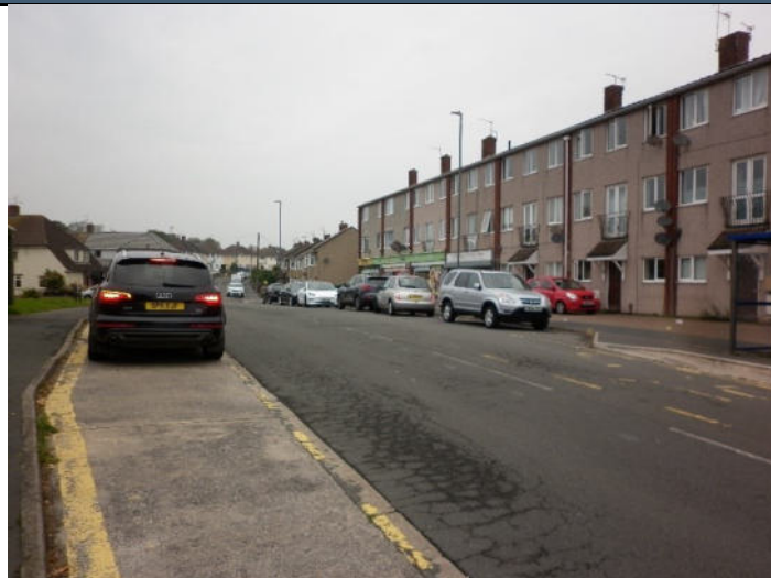
Photo 126: Pound Road (Facing north by Pound Road westbound bus stop)
