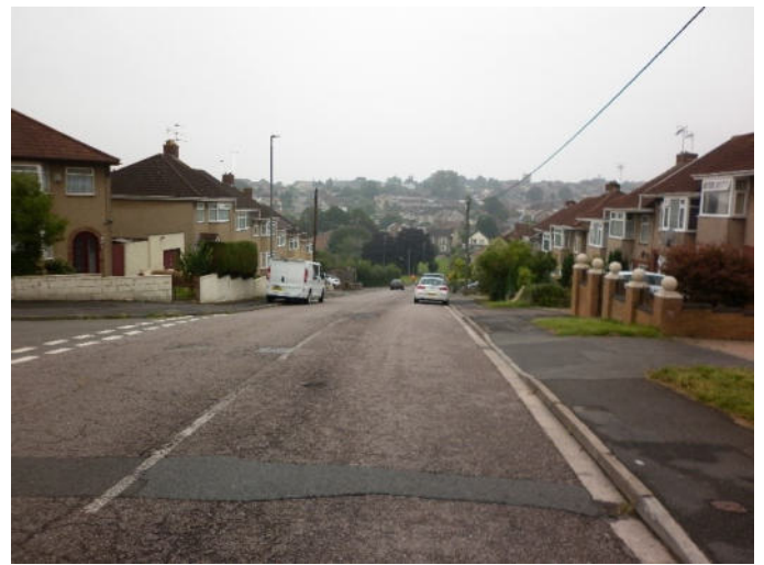
Photo 106: Lees Hill (Facing south by Tyndale Road Junction)
