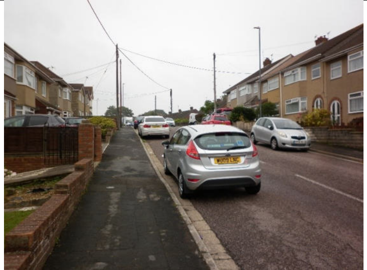
Photo 40: Lees Hill (Facing north by Tyndale Road Junction)
