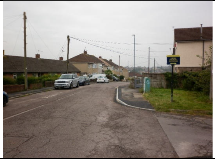
Photo 134: Lees Hill (Facing south by 45A Lees Hill)
