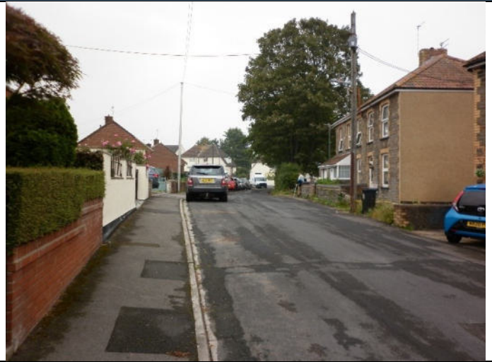
Photo 110: Frys Hill (Facing north by 15 Frys Hill)
