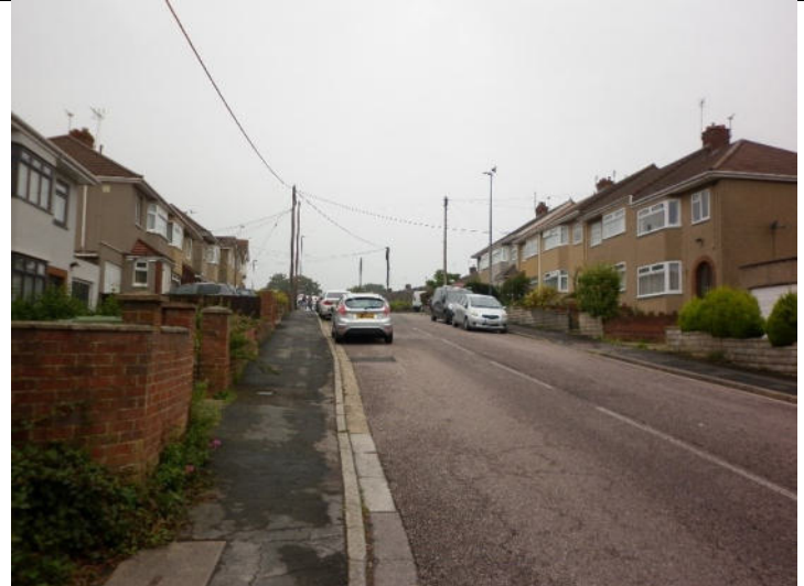
Photo 74: Lees Hill (Facing north by Tyndale Road Junction)
