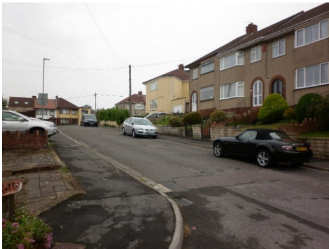
Photo 139: Tyndale Road (Facing west by 10 Tyndale Road)
